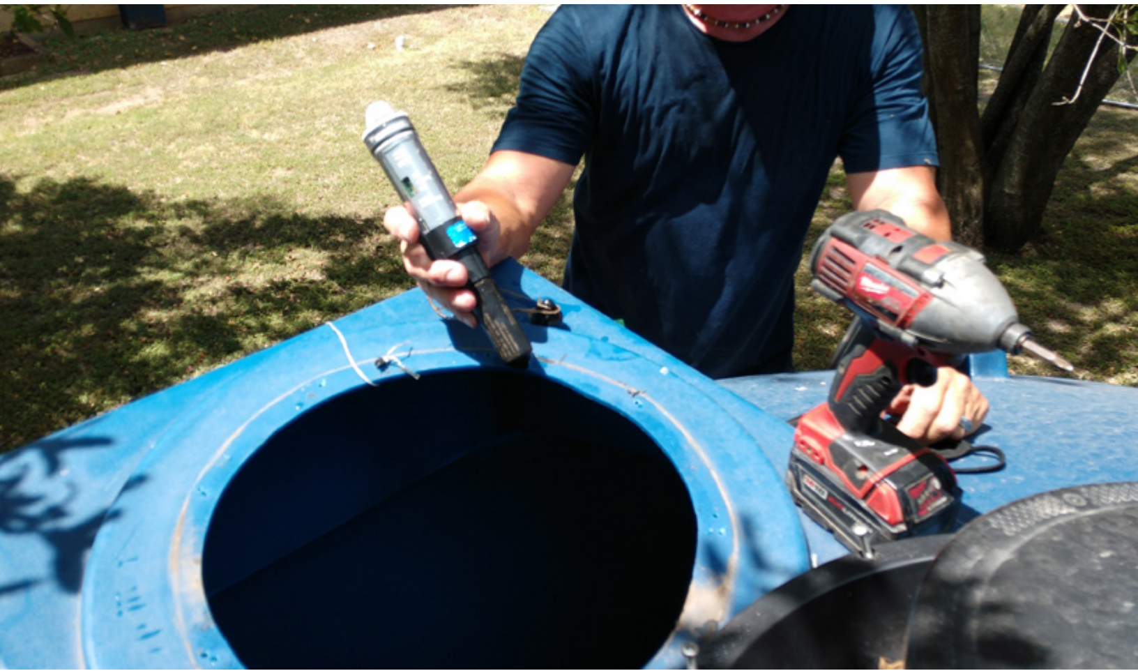
Figure 37. Staff made adjustments to the rainwater collection system
