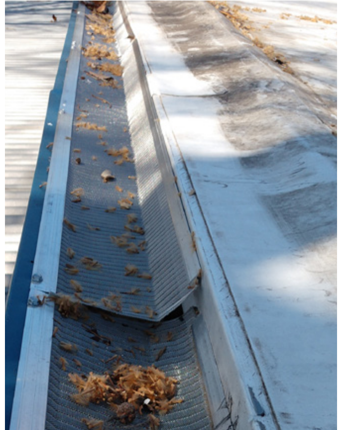
Figure 28. Staff made modifications to the gutter screens.
