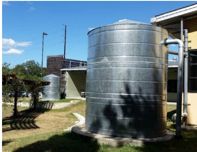
Photos showing connection to roof downspout and outflow to below-ground irrigation system.
