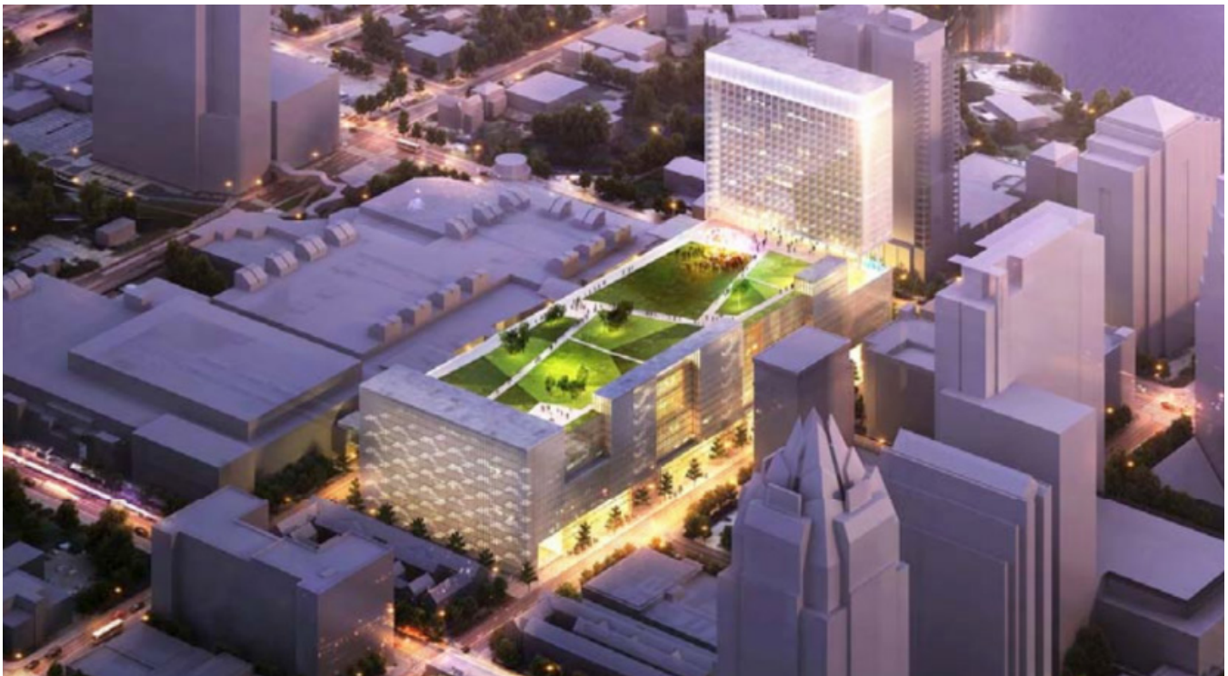
The rendering of the preferred option shows potential green space on the roof deck. (Gensler)
