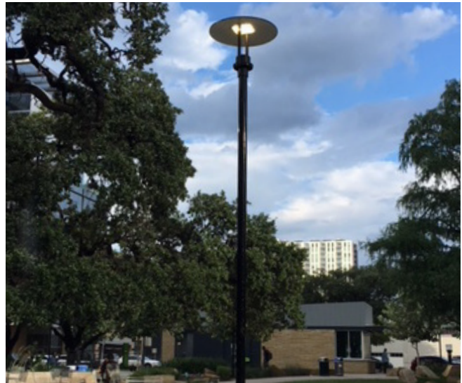
Recently-installed full cut-off pedestrian light fixture at Republic Square (Limbacher Godfrey Architects)
