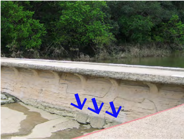
The upstream dam was built in the late 1920s with three openings in it for creek flow. These openings were closed during the 1975 construction of the bypass tunnel. One concept being considered is to install operable openings in the upstream dam.
