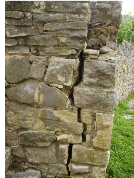
Photo 9: Inside wall of a typical stair.
