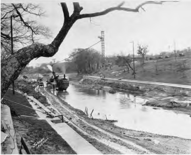
Barton Springs Pool under construction in the 1920s. C01818, Austin History Center, Austin Public Library.
