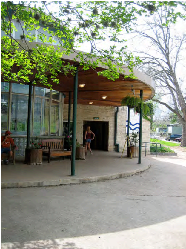
Existing 1947 Bathhouse. Originally, tickets were sold through ticket windows in the glass rotunda.
