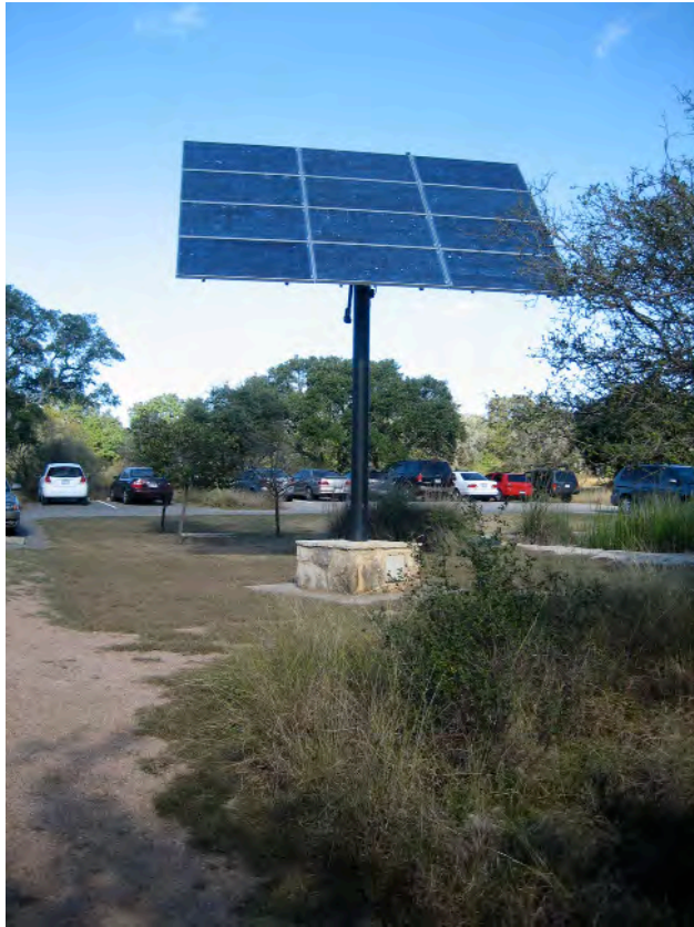
This is a free-standing solar collector at Westcave Preserve. To meaningfully impact energy usage at Barton Springs would require many times more collector area, potentially degrading the park ambiance. But a single collector like this might be enough to power the path lights at the Zilker Ponds.
