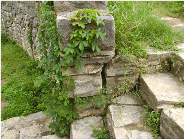
Photo 8: Inside wall of a typical stair.
