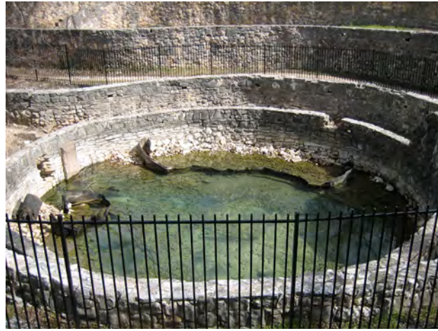
One short-term goal is to repair the walls of the spring vessel. In the same effort, add an operable sluice gate and remove sediment.
