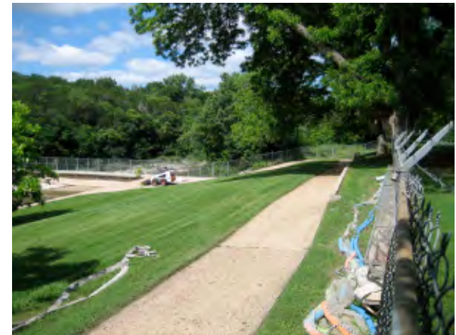
A sliver of grass atop a low retaining wall that is awkward to mow. It is also used for very visible pool equipment storage.
