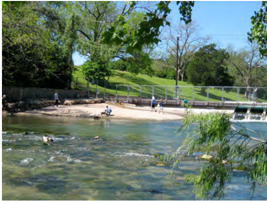
Remove existing concrete and redesign with new stonework for greater comfort and more natural beauty. Using water spilling over the dam, integrate flow into the design to create an attractive “fish ladder” effect.
