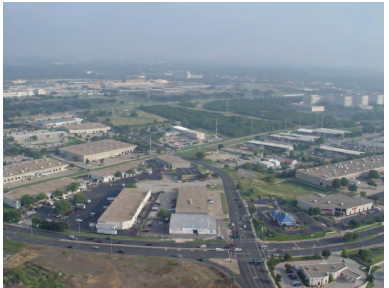
Figure 1.9: Aerial photo of the intersection of Braker Lane and Kramer Lane
