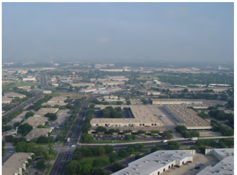
Figure 1.10: Aerial photo of the intersection of Braker Lane and Metric Boulevard
