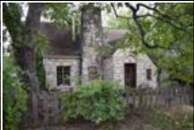
Address: 4815 Avenue H (A) Year Built: 1938 HHM ID: 103146 NR Recommendation: Individually eligible, Within district
