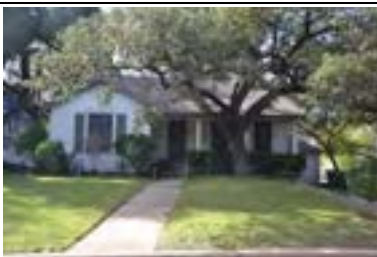
Address: 2844 Shoal Crest Ave (A) Year Built: 1940 HHM ID: 109715 NR Recommendation: Within district
