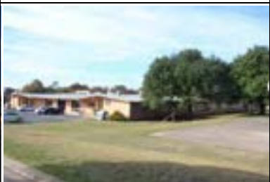
Address: 610 E 45 St Year Built: 1959 HHM ID: 111500 NR Recommendation: Individually eligible, Within district
