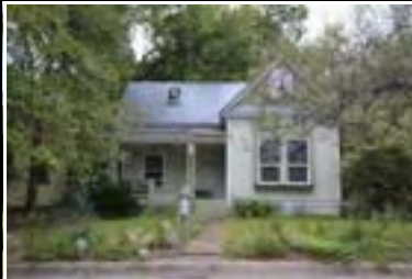
Address: 4526 Avenue C (A) Year Built: 1907 HHM ID: 103706 NR Recommendation: Within district
