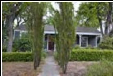
Address: 1710 W 29 St Year Built: 1940 HHM ID: 96559 NR Recommendation: Update previous district listing
