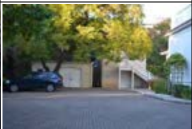
Address: 2310 San Gabriel St (C) Year Built: 1855 HHM ID: 111266 NR Recommendation: Maintain previous listing
