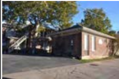
Address: 1900 Pearl St (B) Year Built: 1920 HHM ID: 111209 NR Recommendation: Not eligible
