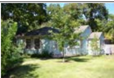
Address: 1702 W 33 St Year Built: 1945 HHM ID: 98444 NR Recommendation: Maintain previous district listing
