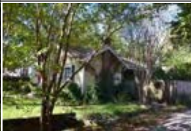
Address: 3710 Tom Green St Year Built: 1930 HHM ID: 105227 NR Recommendation: Within district
