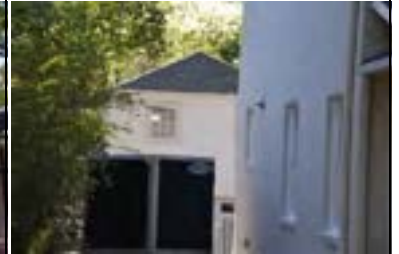
Address: 3105 Harris Blvd (B) Year Built: 1939 HHM ID: 98781 NR Recommendation: Maintain previous district listing
