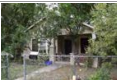
Address: 5000 Rowena St Year Built: 1925 HHM ID: 97841 NR Recommendation: Individually eligible, Within district
