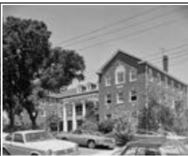
Address: 300 W 29 St Year Built: 1924 HHM ID: 108866 NR Recommendation: Individually eligible
