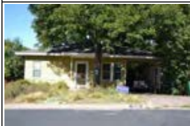
Address: 5006 Rowena St Year Built: 1947 HHM ID: 102693 NR Recommendation: Within district
