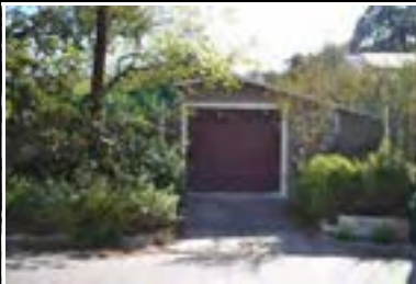
Address: 301 E 35 St (C) Year Built: 1920 HHM ID: 105222 NR Recommendation: Within district
