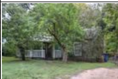
Address: 4515 Avenue D Year Built: 1935 HHM ID: 103931 NR Recommendation: Within district
