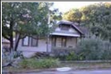
Address: 2202 Longview St Year Built: 1922 HHM ID: 109873 NR Recommendation: Within district
