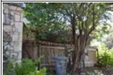
Address: 1104 W M L King Jr Blvd (B) Year Built: 1937 HHM ID: 111104 NR Recommendation: Within district
