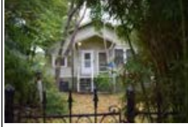
Address: 611 W 31 1/2 St Year Built: 1920 HHM ID: 109179 NR Recommendation: Individually eligible, Within district
