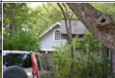
Address: 4706 Rowena St (B) Year Built: 1940 HHM ID: 97908 NR Recommendation: Within district
