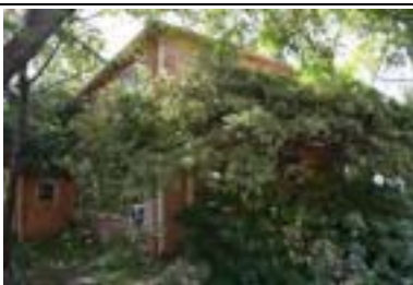
Address: 407 E 38 St (A) Year Built: 1930 HHM ID: 105356 NR Recommendation: Within district
