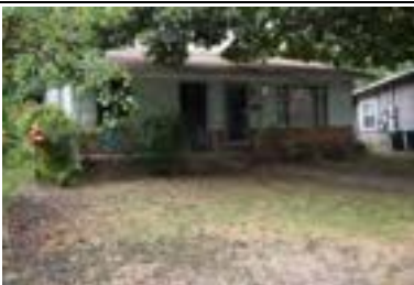
Address: 707 E 46 St (A) Year Built: 1953 HHM ID: 97186 NR Recommendation: Within district
