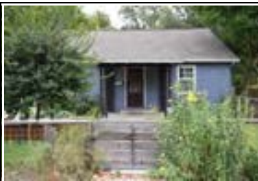
Address: 4607 Avenue D Year Built: 1946 HHM ID: 103874 NR Recommendation: Within district
