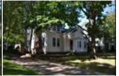
Address: 1515 W 30 St (A) Year Built: 1938 HHM ID: 98891 NR Recommendation: Maintain previous district listing
