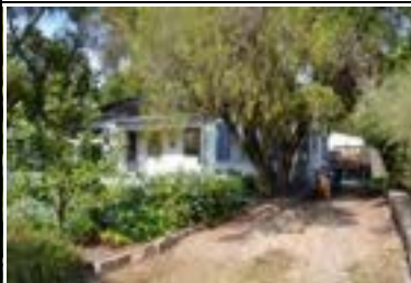
Address: 504 E 46 St (A) Year Built: 1947 HHM ID: 97428 NR Recommendation: Within district
