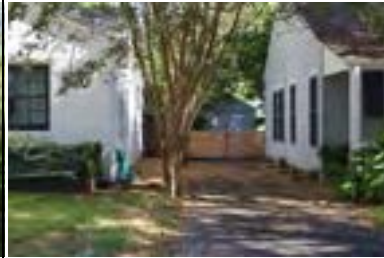
Address: 1514 W 30 St (B) Year Built: 1937 HHM ID: 98895 NR Recommendation: Maintain previous district listing
