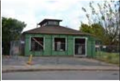
Address: 1700 W 34 St Year Built: 1950 HHM ID: 95855 NR Recommendation: Maintain previous district listing
