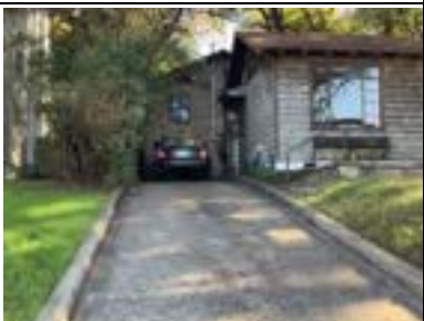
Address: 2307 Shoal Creek Blvd (B) Year Built: 1947 HHM ID: 111390 NR Recommendation: Within district
