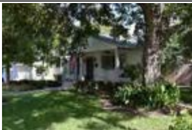
Address: 3301 Bryker Dr Year Built: 1941 HHM ID: 96115 NR Recommendation: Maintain previous district listing
