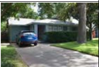
Address: 3305 Bryker Dr Year Built: 1941 HHM ID: 96100 NR Recommendation: Maintain previous district listing
