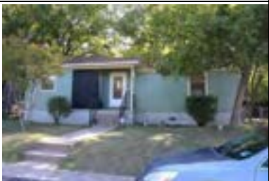
Address: 5003 Rowena St Year Built: 1947 HHM ID: 102735 NR Recommendation: Within district
