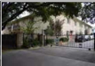
Address: 2711 Rio Grande St Year Built: 1970 HHM ID: 110434 NR Recommendation: Individually eligible
