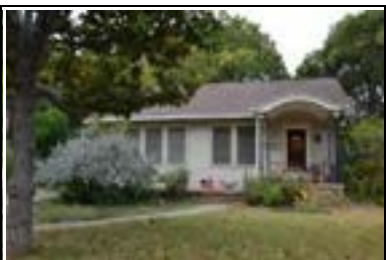
Address: 4814 Red River St Year Built: 1929 HHM ID: 96771 NR Recommendation: Within district
