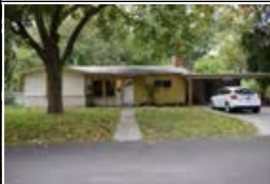
Address: 4600 Avenue D Year Built: 1952 HHM ID: 103831 NR Recommendation: Within district
