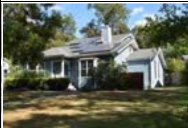
Address: 3207 Bryker Dr Year Built: 1940 HHM ID: 96147 NR Recommendation: Maintain previous district listing
