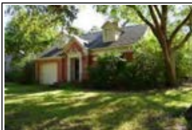
Address: 2901 Glenview Ave Year Built: 1941 HHM ID: 98280 NR Recommendation: Maintain previous district listing
