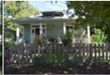
Address: 204 E 35 St Year Built: 1917 HHM ID: 105281 NR Recommendation: Individually eligible, Within district
