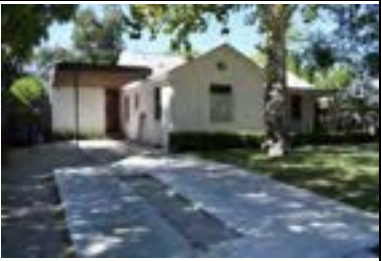
Address: 3004 Kerbey Ln Year Built: 1939 HHM ID: 98497 NR Recommendation: Maintain previous district listing
