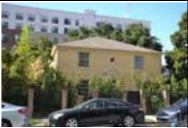
Address: 2210 Nueces St (A) Year Built: 1941 HHM ID: 111327 NR Recommendation: Individually eligible
