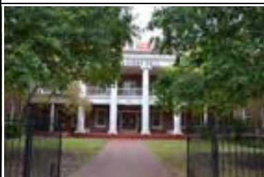
Address: 300 W 29 St Year Built: 1924 HHM ID: 108866 NR Recommendation: Individually eligible
