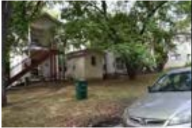
Address: 3306 Tom Green St (B) Year Built: 1974 HHM ID: 107694 NR Recommendation: Within district
