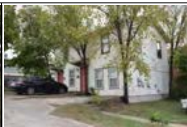
Address: 3305 Grooms St (B) Year Built: 1948 HHM ID: 107775 NR Recommendation: Within district
