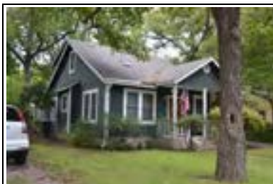
Address: 4510 Avenue D (A) Year Built: 1940 HHM ID: 103878 NR Recommendation: Within district
