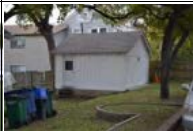
Address: 201 E 33 St (B) Year Built: 1925 HHM ID: 107760 NR Recommendation: Within district
