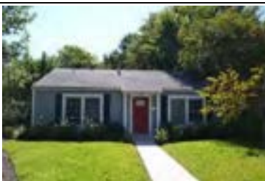
Address: 1701 W 33 St Year Built: 1948 HHM ID: 98442 NR Recommendation: Maintain previous district listing
