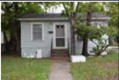
Address: 316 W 34 St (A) Year Built: 1948 HHM ID: 107628 NR Recommendation: Within district
