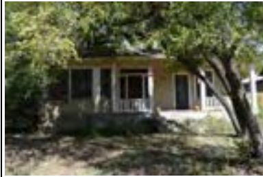
Address: 200 E 35 St Year Built: 1917 HHM ID: 105289 NR Recommendation: Individually eligible, Within district
