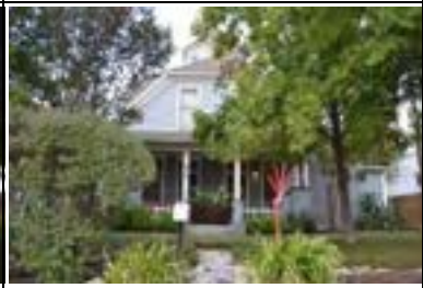
Address: 200 E 32 St Year Built: 1894 HHM ID: 107896 NR Recommendation: Individually eligible, Within district
