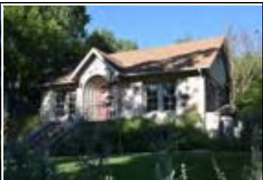
Address: 3104 Harris Blvd Year Built: 1940 HHM ID: 98779 NR Recommendation: Maintain previous district listing
