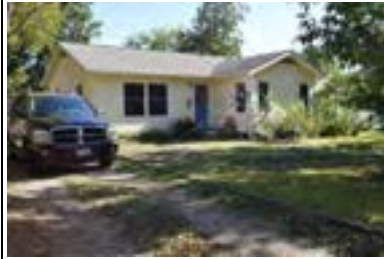
Address: 4709 Eilers Ave (A) Year Built: 1949 HHM ID: 104829 NR Recommendation: Within district
