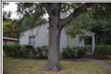
Address: 4605 Caswell Ave (A) Year Built: 1939 HHM ID: 97024 NR Recommendation: Within district
