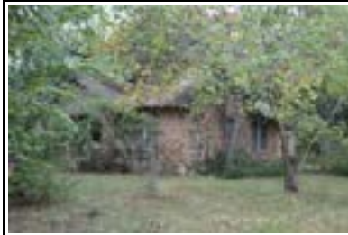
Address: 4612 Red River St (A) Year Built: 1930 HHM ID: 97094 NR Recommendation: Individually eligible, Within district
