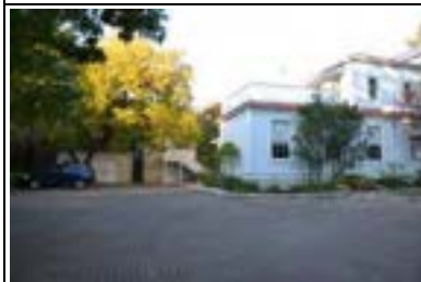
Address: 2310 San Gabriel St (B) Year Built: 1855 HHM ID: 111262 NR Recommendation: Maintain previous listing
