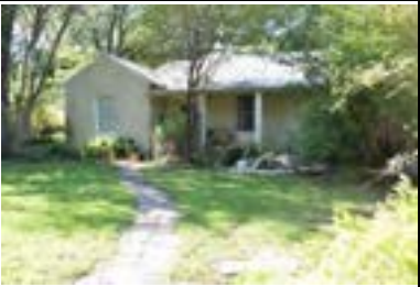
Address: 3000 Kerbey Ln Year Built: 1937 HHM ID: 98507 NR Recommendation: Maintain previous district listing
