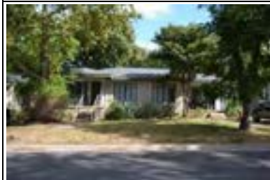
Address: 1908 W 33 St Year Built: 1949 HHM ID: 95961 NR Recommendation: Maintain previous district listing
