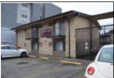
Address: 2610 Salado St Year Built: 1966 HHM ID: 110580 NR Recommendation: Not eligible
