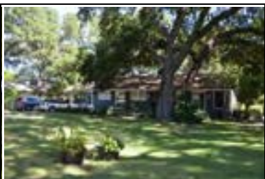
Address: 2907 Oakhurst Ave Year Built: 1951 HHM ID: 99126 NR Recommendation: Add to listed district
