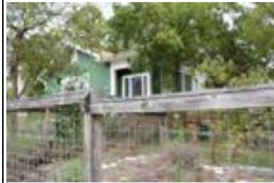
Address: 620 W 35 St (A) Year Built: 1922 HHM ID: 108090 NR Recommendation: Individually eligible, Within district
