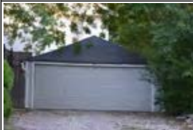
Address: 3202 Glenview Ave (B) Year Built: 1950 HHM ID: 98144 NR Recommendation: Update previous district listing
