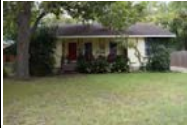
Address: 807 E 49 St (A) Year Built: 1949 HHM ID: 96825 NR Recommendation: Within district
