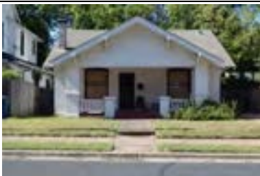
Address: 3310 Jefferson St Year Built: 1920 HHM ID: 98452 NR Recommendation: Maintain previous district listing
