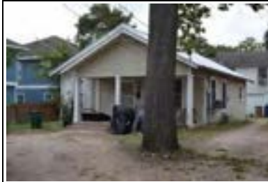
Address: 611 W 37 St (A) Year Built: 1930 HHM ID: 108027 NR Recommendation: Within district
