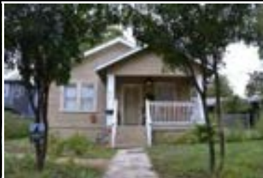
Address: 4810 Avenue H (A) Year Built: 1925 HHM ID: 104308 NR Recommendation: Within district
