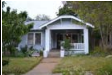
Address: 2838 Pearl St Year Built: 1930 HHM ID: 109330 NR Recommendation: Individually eligible, Within district
