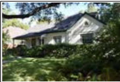
Address: 1514 W 29 St Year Built: 1938 HHM ID: 98876 NR Recommendation: Maintain previous district listing
