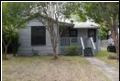
Address: 5006 Eilers Ave (A) Year Built: 1947 HHM ID: 96922 NR Recommendation: Within district
