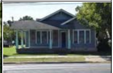
Address: 305 E 38 St (A) Year Built: 1925 HHM ID: 105323 NR Recommendation: Individually eligible, Within district
