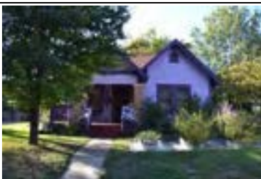
Address: 4800 Avenue G (A) Year Built: 1932 HHM ID: 102898 NR Recommendation: Within district
