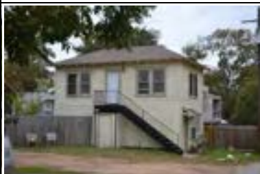
Address: 1102 W 22 St (B) Year Built: 1922 HHM ID: 110182 NR Recommendation: Within district
