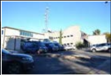
Address: 906 W M L King Jr Blvd Year Built: 1965 HHM ID: 111202 NR Recommendation: Not eligible
