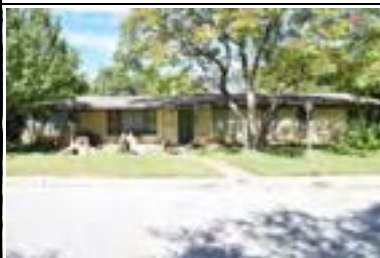
Address: 612 E 48 St Year Built: 1953 HHM ID: 104802 NR Recommendation: Individually eligible, Within district
