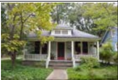
Address: 4518 Avenue C Year Built: 1910 HHM ID: 103775 NR Recommendation: Individually eligible, Within district
