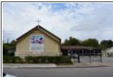
Address: 5002 Caswell Ave Year Built: 1942 HHM ID: 96744 NR Recommendation: Within district
