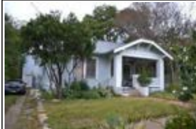
Address: 2838 Pearl St Year Built: 1930 HHM ID: 109330 NR Recommendation: Individually eligible, Within district
