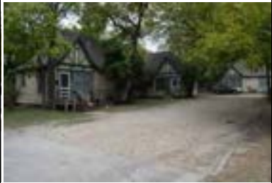
Address: 404 W 34 St (A) Year Built: 1936 HHM ID: 107587 NR Recommendation: Individually eligible, Within district
