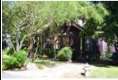
Address: 1516 W 31 St Year Built: 1939 HHM ID: 98994 NR Recommendation: Update previous district listing
