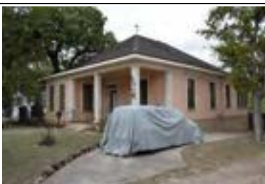
Address: 606 W 35 St Year Built: 1915 HHM ID: 108064 NR Recommendation: Individually eligible, Within district
