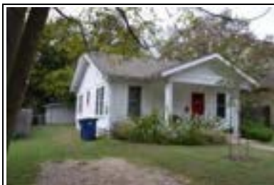
Address: 4530 Avenue F (A) Year Built: 1930 HHM ID: 104070 NR Recommendation: Within district
