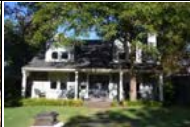
Address: 3102 Glenview Ave Year Built: 1938 HHM ID: 98191 NR Recommendation: Maintain previous district listing
