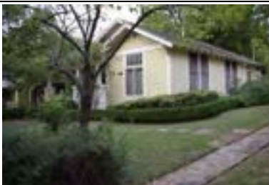
Address: 4714 Avenue G Year Built: 1925 HHM ID: 102953 NR Recommendation: Individually eligible, Within district
