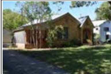
Address: 3006 Kerbey Ln (A) Year Built: 1939 HHM ID: 98486 NR Recommendation: Maintain previous district listing
