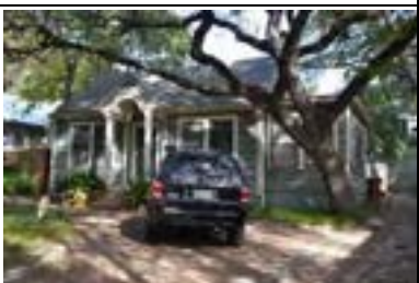
Address: 2839 Shoal Crest Ave Year Built: 1930 HHM ID: 109737 NR Recommendation: Within district
