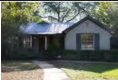
Address: 2907 Glenview Ave Year Built: 1938 HHM ID: 98254 NR Recommendation: Maintain previous district listing
