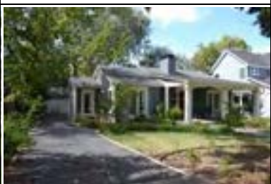
Address: 3304 Bryker Dr (A) Year Built: 1940 HHM ID: 96105 NR Recommendation: Maintain previous district listing
