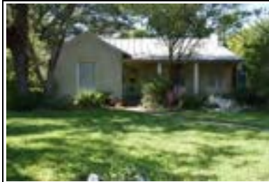
Address: 3000 Kerbey Ln Year Built: 1937 HHM ID: 98507 NR Recommendation: Maintain previous district listing
