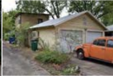
Address: 5000 Duval St (B) Year Built: 1935 HHM ID: 97830 NR Recommendation: Within district
