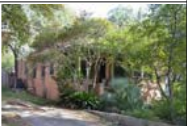
Address: 2833 Shoal Crest Ave Year Built: 1931 HHM ID: 109780 NR Recommendation: Within district
