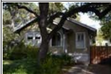
Address: 2841 Shoal Crest Ave Year Built: 1928 HHM ID: 109733 NR Recommendation: Within district
