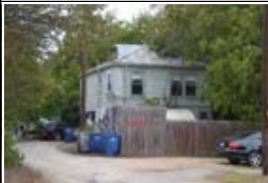
Address: 4504 Red River St (B) Year Built: 1955 HHM ID: 97247 NR Recommendation: Within district
