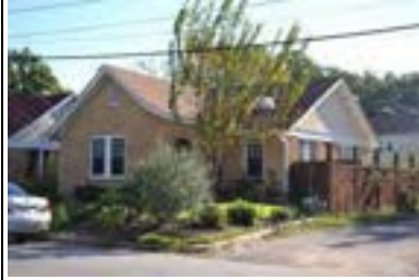
Address: 3405 B Tom Green St Year Built: 1930 HHM ID: 105095 NR Recommendation: Within district
