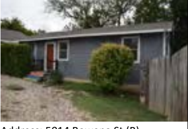
Address: 5014 Rowena St (B) Year Built: 1950 HHM ID: 97832 NR Recommendation: Within district
