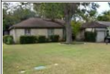
Address: 1905 W 33 St Year Built: 1959 HHM ID: 95983 NR Recommendation: Maintain previous district listing
