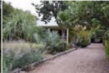
Address: 3206 Oakmont Blvd Year Built: 1947 HHM ID: 96488 NR Recommendation: Maintain previous district listing
