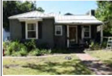
Address: 1515 W 31 St Year Built: 1938 HHM ID: 98991 NR Recommendation: Maintain previous district listing
