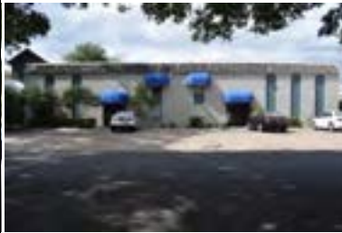
Address: 4412 Avenue A Year Built: 1967 HHM ID: 103326 NR Recommendation: Within district
