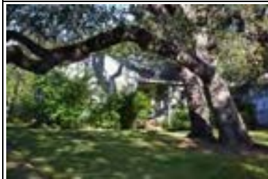
Address: 3004 Glenview Ave Year Built: 1938 HHM ID: 98217 NR Recommendation: Individually eligible, Maintain previous district listing
