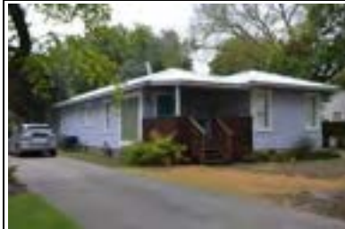
Address: 3211 Beverly Rd (A) Year Built: 1948 HHM ID: 96225 NR Recommendation: Update previous district listing
