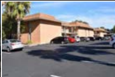
Address: 302 W 38 St (A) Year Built: 1968 HHM ID: 105130 NR Recommendation: Not eligible
