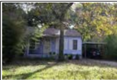
Address: 4517 Avenue D Year Built: 1946 HHM ID: 103923 NR Recommendation: Within district
