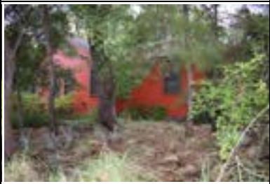
Address: 3201 Bryker Dr Year Built: 1941 HHM ID: 96173 NR Recommendation: Maintain previous district listing
