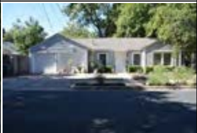
Address: 3304 Jefferson St (B) Year Built: 1949 HHM ID: 98443 NR Recommendation: Update previous district listing
