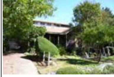
Address: 1516 W 31 St Year Built: 1939 HHM ID: 98994 NR Recommendation: Update previous district listing
