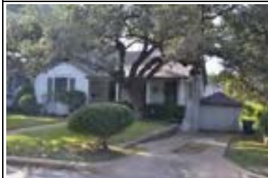
Address: 2844 Shoal Crest Ave (B) Year Built: 1940 HHM ID: 109721 NR Recommendation: Within district
