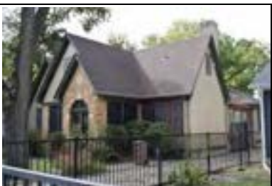
Address: 3506 Duval St Year Built: 1927 HHM ID: 105365 NR Recommendation: Within district
