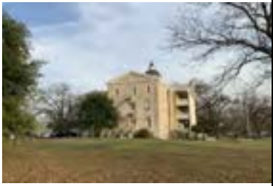
Address: 4110 Guadalupe St (A) Year Built: 1857 HHM ID: 113311 NR Recommendation: Maintain previous listing, Within district
