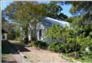
Address: 301 E 35 St (A) Year Built: 1920 HHM ID: 105212 NR Recommendation: Individually eligible, Within district
