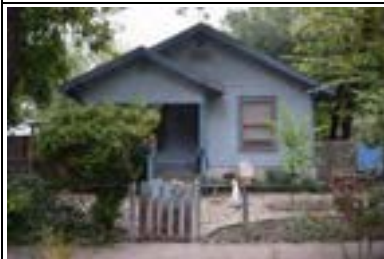
Address: 4504 Avenue C Year Built: 1925 HHM ID: 103731 NR Recommendation: Individually eligible, Within district
