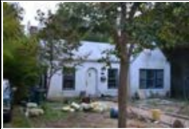
Address: 403 E 32 St Year Built: 1934 HHM ID: 107992 NR Recommendation: Individually eligible, Within district
