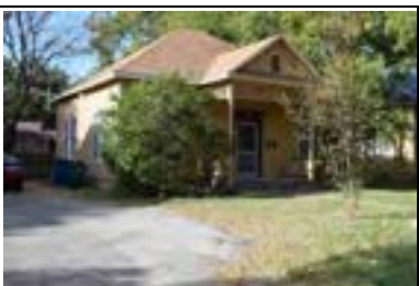
Address: 3102 King St (A) Year Built: 1918 HHM ID: 109707 NR Recommendation: Individually eligible, Within district
