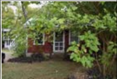
Address: 310 W 34 St (A) Year Built: 1948 HHM ID: 107657 NR Recommendation: Within district
