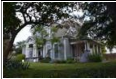
Address: 200 E 32 St Year Built: 1894 HHM ID: 107896 NR Recommendation: Individually eligible, Within district
