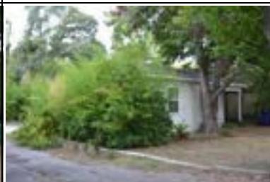
Address: 3306 Grooms St (A) Year Built: 1939 HHM ID: 107583 NR Recommendation: Within district
