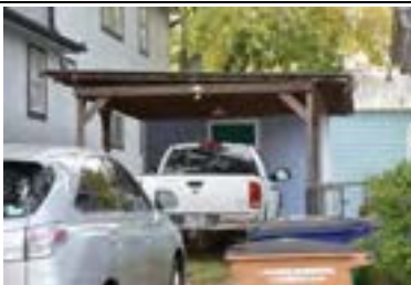
Address: 609 W 35 St (B) Year Built: 1930 HHM ID: 108082 NR Recommendation: Within district
