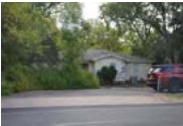
Address: 3404 Glenview Ave Year Built: 1950 HHM ID: 95848 NR Recommendation: Maintain previous district listing
