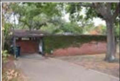
Address: 1111 W 31 St Year Built: 1953 HHM ID: 96596 NR Recommendation: Individually eligible
