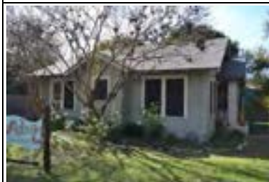
Address: 913 W 29 St Year Built: 1928 HHM ID: 109635 NR Recommendation: Individually eligible, Within district
