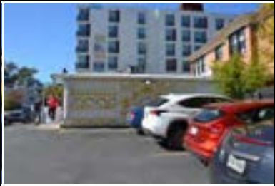
Address: 600 W M L King Jr Blvd Year Built: 1969 HHM ID: 111314 NR Recommendation: Not eligible
