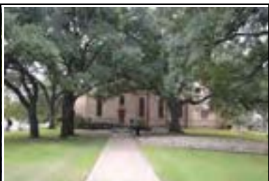
Address: 100 E 27 St (B) Year Built: 1941 HHM ID: 108765 NR Recommendation: Individually eligible, Within district
