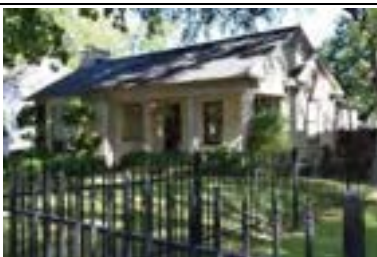
Address: 1504 W 29 St (A) Year Built: 1938 HHM ID: 98854 NR Recommendation: Maintain previous district listing
