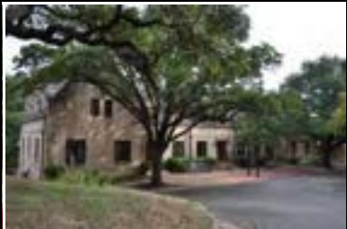
Address: 100 E 27 St (E) Year Built: 1945 HHM ID: 108786 NR Recommendation: Within district
