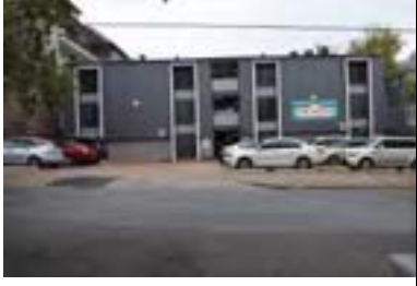
Address: 2704 Salado St Year Built: 1972 HHM ID: 110590 NR Recommendation: Not eligible
