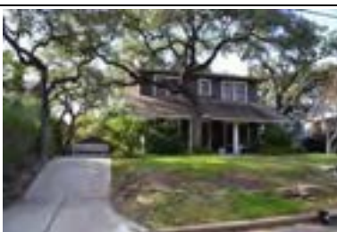
Address: 2840 Shoal Crest Ave (A) Year Built: 1932 HHM ID: 109754 NR Recommendation: Within district
