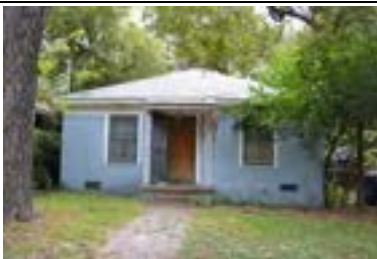
Address: 4511 Avenue G (A) Year Built: 1930 HHM ID: 103082 NR Recommendation: Within district
