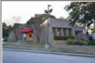
Address: 1601 W 35 St Year Built: 1974 HHM ID: 111519 NR Recommendation: Individually eligible
