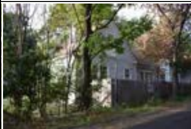
Address: 708 W 32 St (A) Year Built: 1937 HHM ID: 108312 NR Recommendation: Within district
