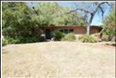
Address: 3012 Oakhurst Ave Year Built: 1957 HHM ID: 99084 NR Recommendation: Add to listed district
