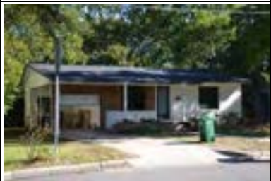
Address: 3205 Kerbey Ln Year Built: 1957 HHM ID: 98591 NR Recommendation: Maintain previous district listing
