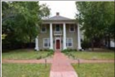
Address: 3005 Washington Sq Year Built: 1930 HHM ID: 109070 NR Recommendation: Individually eligible, Within district
