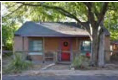
Address: 5002 Avenue F (A) Year Built: 1947 HHM ID: 102795 NR Recommendation: Within district
