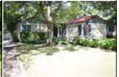
Address: 3006 Beverly Rd Year Built: 1941 HHM ID: 98321 NR Recommendation: Maintain previous district listing
