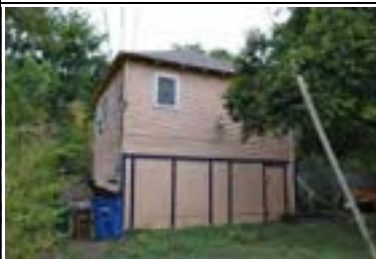
Address: 305 E 47th St (B) Year Built: 1930 HHM ID: 97637 NR Recommendation: Within district
