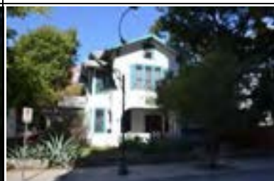
Address: 510 W 23 St Year Built: 1920 HHM ID: 111333 NR Recommendation: Individually eligible
