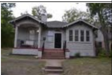
Address: 805 W 28 1/2 St (A) Year Built: 1924 HHM ID: 109316 NR Recommendation: Individually eligible, Within district
