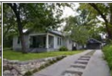
Address: 4807 Avenue F (A) Year Built: 1933 HHM ID: 97765 NR Recommendation: Individually eligible, Within district
