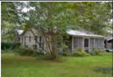
Address: 4806 Rowena St Year Built: 1945 HHM ID: 97866 NR Recommendation: Within district
