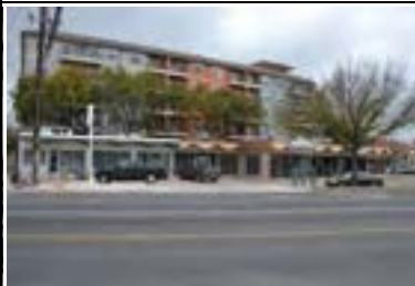
Address: 605 W 29 St Year Built: 1962 HHM ID: 109032 NR Recommendation: Individually eligible, Within district
