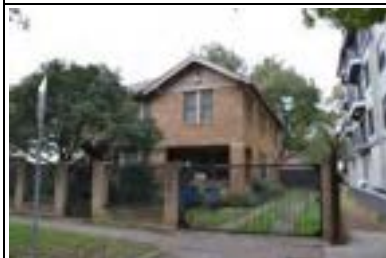
Address: 910 W 22 1/2 St Year Built: 1932 HHM ID: 110199 NR Recommendation: Individually eligible
