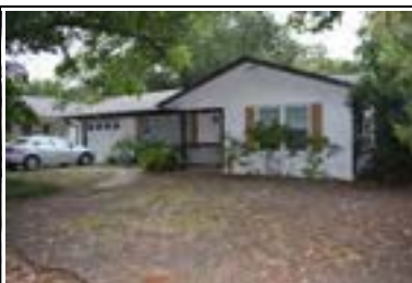
Address: 4603 Caswell Ave Year Built: 1960 HHM ID: 97021 NR Recommendation: Within district
