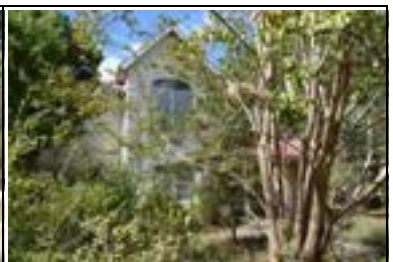
Address: 3402 Glenview Ave Year Built: 1965 HHM ID: 96046 NR Recommendation: Maintain previous district listing
