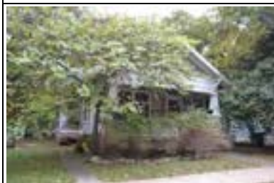
Address: 907 W 22 1/2 St Year Built: 1932 HHM ID: 110214 NR Recommendation: Individually eligible
