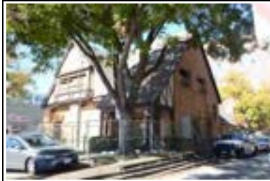
Address: 506 W M L King Jr Blvd Year Built: 1932 HHM ID: 111316 NR Recommendation: Individually eligible
