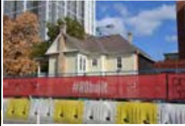
Address: 611 W 22 St Year Built: 1907 HHM ID: 111569 NR Recommendation: Individually eligible
