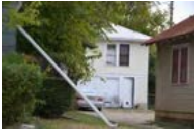
Address: 1905 David St (B) Year Built: 1938 HHM ID: 110393 NR Recommendation: Within district
