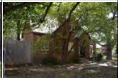
Address: 4415 Avenue A (A) Year Built: 1936 HHM ID: 103316 NR Recommendation: Maintain previous listing, Within district
