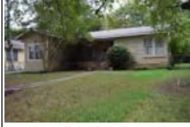
Address: 1704 W 30 St Year Built: 1951 HHM ID: 96580 NR Recommendation: Update previous district listing
