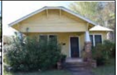
Address: 107 E 38 St Year Built: 1927 HHM ID: 105254 NR Recommendation: Individually eligible, Within district
