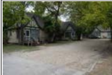
Address: 404 W 34 St (B) Year Built: 1936 HHM ID: 107594 NR Recommendation: Individually eligible, Within district
