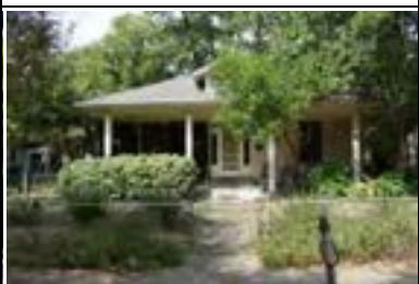
Address: 4514 Caswell Ave Year Built: 1919 HHM ID: 97275 NR Recommendation: Within district
