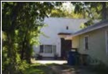
Address: 4903 Avenue F (B) Year Built: 1950 HHM ID: 102772 NR Recommendation: Within district
