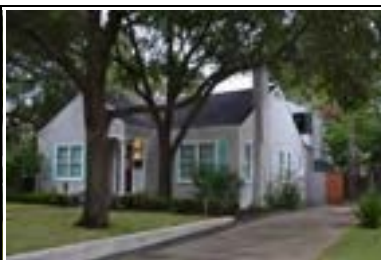
Address: 3204 Bryker Dr Year Built: 1940 HHM ID: 96162 NR Recommendation: Maintain previous district listing
