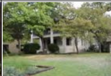
Address: 614 W 32 St Year Built: 1901 HHM ID: 109437 NR Recommendation: Individually eligible, Within district
