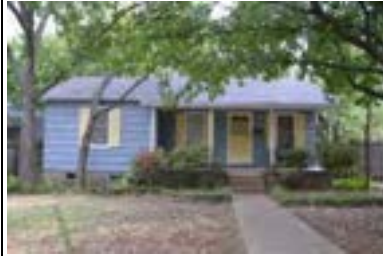
Address: 3006 Funston St Year Built: 1949 HHM ID: 96388 NR Recommendation: Maintain previous district listing
