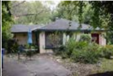
Address: 4611 Avenue D Year Built: 1946 HHM ID: 103851 NR Recommendation: Within district
