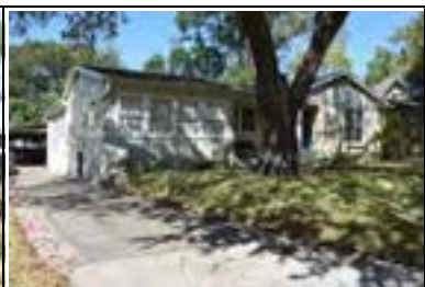
Address: 3004 Bryker Dr Year Built: 1941 HHM ID: 98422 NR Recommendation: Maintain previous district listing
