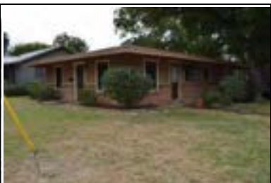
Address: 701 E 46 St (A) Year Built: 1953 HHM ID: 97215 NR Recommendation: Within district
