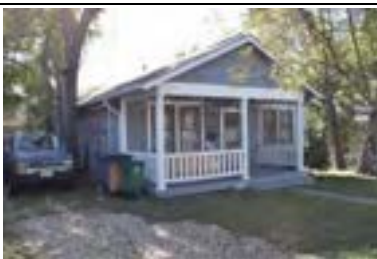
Address: 407 W 37 St Year Built: 1930 HHM ID: 107334 NR Recommendation: Individually eligible, Within district
