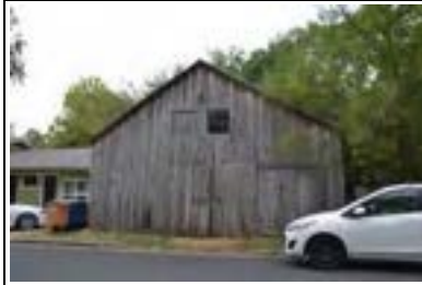
Address: 4529 Avenue G (C) Year Built: 1925 HHM ID: 103053 NR Recommendation: Within district
