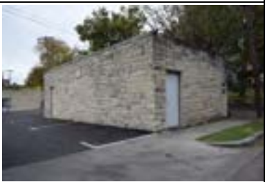
Address: 2934 Guadalupe St (B) Year Built: 1938 HHM ID: 108715 NR Recommendation: Within district
