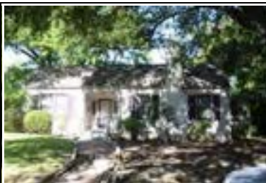
Address: 1522 W 32 St Year Built: 1938 HHM ID: 98519 NR Recommendation: Individually eligible, Maintain previous district listing
