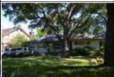
Address: 3001 Oakhurst Ave Year Built: 1952 HHM ID: 99145 NR Recommendation: Add to listed district
