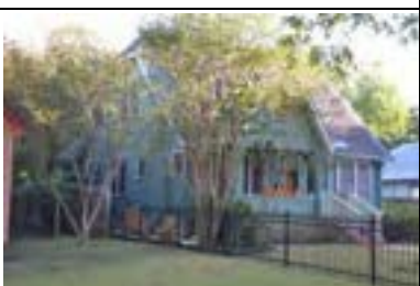
Address: 402 E 35 St (A) Year Built: 1930 HHM ID: 104967 NR Recommendation: Within district
