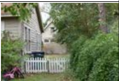
Address: 710 W 35 St (B) Year Built: 1932 HHM ID: 108148 NR Recommendation: Within district
