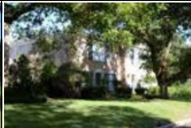
Address: 2904 Glenview Ave Year Built: 1973 HHM ID: 98245 NR Recommendation: Update previous district listing
