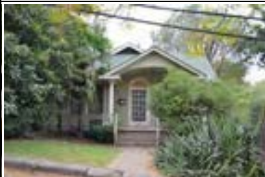
Address: 2902 Hemphill Park (A) Year Built: 1930 HHM ID: 108909 NR Recommendation: Individually eligible
