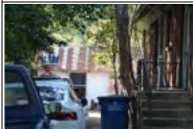
Address: 2832 Shoal Crest Ave (B) Year Built: 1940 HHM ID: 109602 NR Recommendation: Within district
