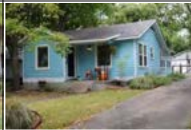
Address: 508 E 49 St (A) Year Built: 1951 HHM ID: 97751 NR Recommendation: Within district
