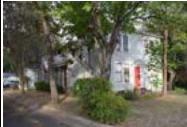
Address: 706 W 32 St (A) Year Built: 1930 HHM ID: 108318 NR Recommendation: Within district
