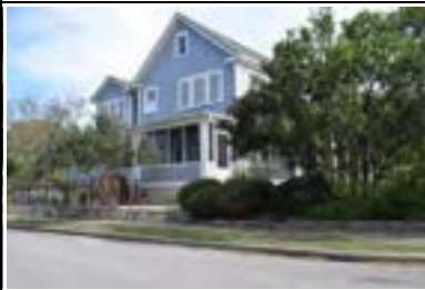
Address: 810 W 31 St (A) Year Built: 1915 HHM ID: 109573 NR Recommendation: Individually eligible, Within district
