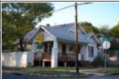
Address: 2200 Longview St Year Built: 1922 HHM ID: 109872 NR Recommendation: Individually eligible, Within district
