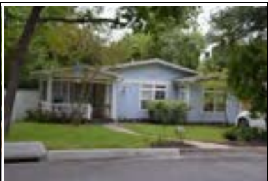
Address: 1901 W 30 St Year Built: 1951 HHM ID: 96397 NR Recommendation: Maintain previous district listing
