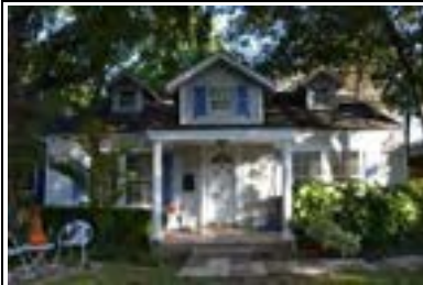
Address: 3307 Glenview Ave Year Built: 1938 HHM ID: 98099 NR Recommendation: Maintain previous district listing
