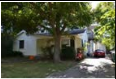
Address: 609 Fairfield Ln (A) Year Built: 1950 HHM ID: 104788 NR Recommendation: Within district
