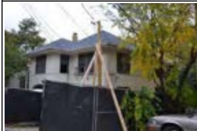
Address: 2807 Hemphill Park Year Built: 1930 HHM ID: 108894 NR Recommendation: Individually eligible
