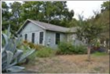
Address: 4800 A Red River Year Built: 1945 HHM ID: 96826 NR Recommendation: Within district
