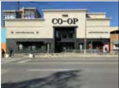
Address: 2266 Guadalupe St (A) Year Built: 1958 HHM ID: 110840 NR Recommendation: Within district
