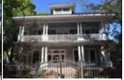
Address: 612 W 22 St Year Built: 1905 HHM ID: 111028 NR Recommendation: Individually eligible
