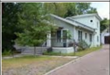
Address: 512 E 49 St (A) Year Built: 1925 HHM ID: 97763 NR Recommendation: Within district
