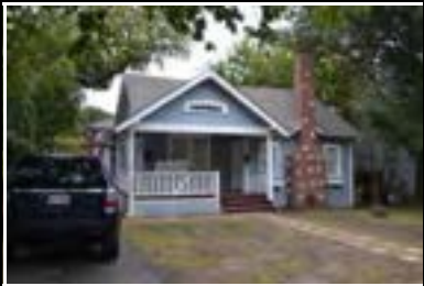
Address: 1109 W 22 1/2 St Year Built: 1927 HHM ID: 110030 NR Recommendation: Individually eligible, Within district
