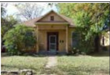
Address: 3102 King St (A) Year Built: 1918 HHM ID: 109707 NR Recommendation: Individually eligible, Within district
