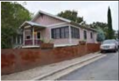
Address: 609 W 31 1/2 St Year Built: 1920 HHM ID: 109148 NR Recommendation: Individually eligible, Within district
