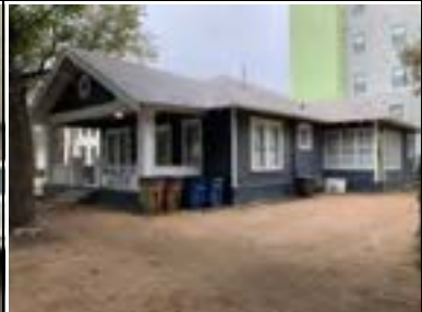
Address: 604 W 25 St Year Built: 1920 HHM ID: 110625 NR Recommendation: Individually eligible
