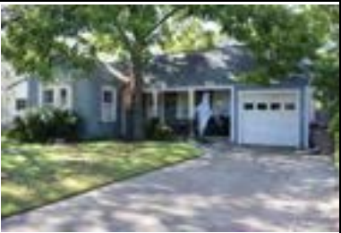
Address: 2906 Kerbey Ln Year Built: 1938 HHM ID: 98526 NR Recommendation: Maintain previous district listing
