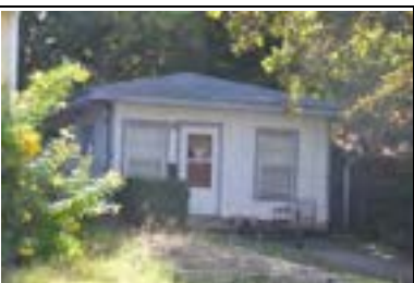
Address: 5007 Rowena St Year Built: 1948 HHM ID: 102731 NR Recommendation: Within district
