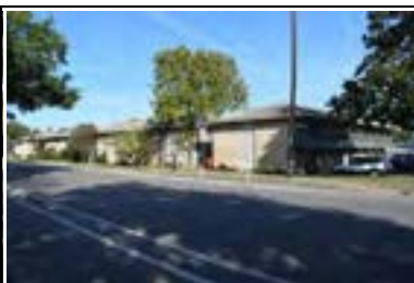
Address: 3403 Speedway (D) Year Built: 1959 HHM ID: 107421 NR Recommendation: Within district
