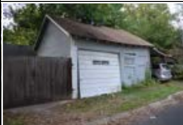
Address: 708 W 32 St (B) Year Built: 1937 HHM ID: 108313 NR Recommendation: Within district
