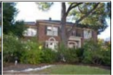
Address: 1900 Pearl St (A) Year Built: 1920 HHM ID: 111187 NR Recommendation: Individually eligible
