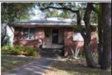
Address: 2835 Shoal Crest Ave Year Built: 1930 HHM ID: 109765 NR Recommendation: Within district
