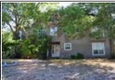
Address: 3001 Beverly Rd Year Built: 1948 HHM ID: 98290 NR Recommendation: Maintain previous district listing
