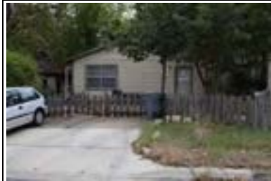
Address: 4815 Avenue H (B) Year Built: 1938 HHM ID: 103156 NR Recommendation: Within district
