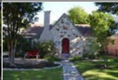
Address: 1510 W 29 St Year Built: 1937 HHM ID: 98862 NR Recommendation: Maintain previous district listing
