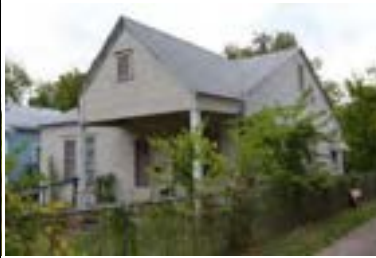
Address: 611 W 35 St (A) Year Built: 1938 HHM ID: 108087 NR Recommendation: Within district
