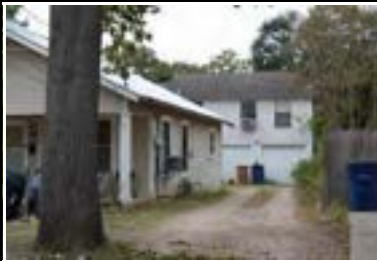
Address: 611 W 37 St (B) Year Built: 1938 HHM ID: 108033 NR Recommendation: Within district
