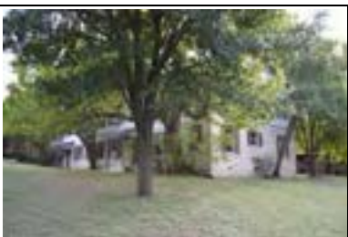
Address: 301 A E 33 St Year Built: 1949 HHM ID: 107727 NR Recommendation: Within district
