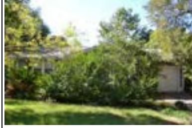
Address: 1805 W 30 St Year Built: 1957 HHM ID: 98310 NR Recommendation: Update previous district listing
