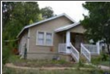
Address: 4810 Avenue H (A) Year Built: 1925 HHM ID: 104308 NR Recommendation: Within district
