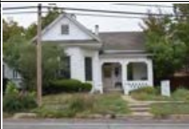
Address: 200 E 30 St Year Built: 1907 HHM ID: 108493 NR Recommendation: Individually eligible, Within district
