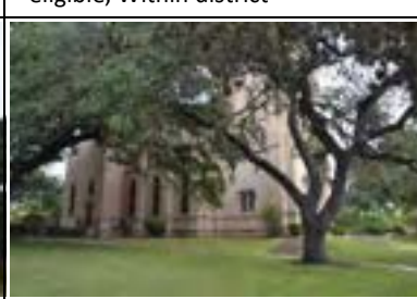
Address: 100 E 27 St (B) Year Built: 1941 HHM ID: 108765 NR Recommendation: Individually eligible, Within district
