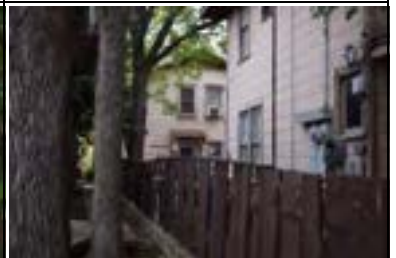
Address: 204 E 30 St (B) Year Built: 1925 HHM ID: 108479 NR Recommendation: Within district
