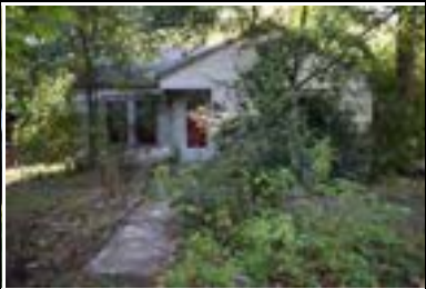
Address: 4533 Avenue H (A) Year Built: 1939 HHM ID: 104515 NR Recommendation: Within district
