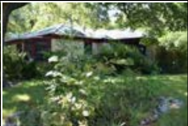
Address: 615 E 48 St (A) Year Built: 1949 HHM ID: 104795 NR Recommendation: Within district
