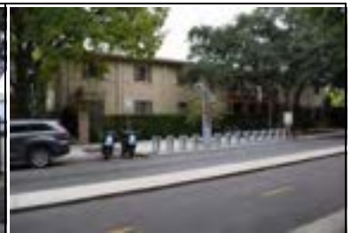
Address: 2711 Rio Grande St Year Built: 1970 HHM ID: 110434 NR Recommendation: Individually eligible
