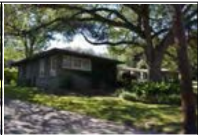
Address: 1303 Belmont Pkwy Year Built: 1955 HHM ID: 99159 NR Recommendation: Add to listed district
