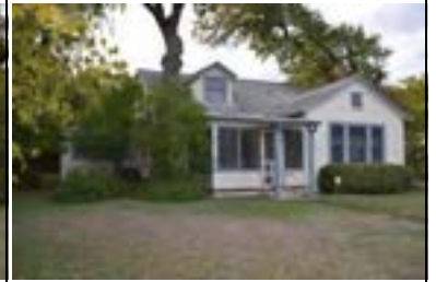
Address: 3114 West Ave Year Built: 1922 HHM ID: 108311 NR Recommendation: Within district
