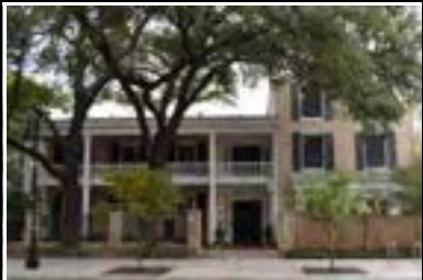
Address: 2620 Rio Grande St (A) Year Built: 1871 HHM ID: 110443 NR Recommendation: Individually eligible
