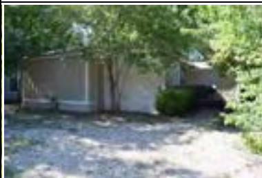
Address: 3306 Jefferson St Year Built: 1955 HHM ID: 98448 NR Recommendation: Maintain previous district listing
