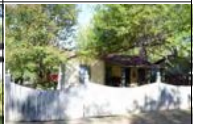
Address: 5014 Avenue F (A) Year Built: 1941 HHM ID: 102705 NR Recommendation: Within district
