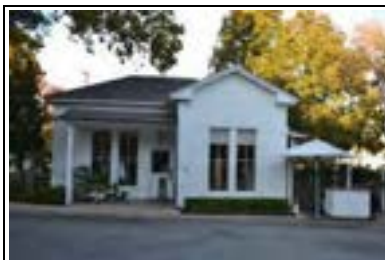
Address: 1515 B W 35 St (B) Year Built: 1920 HHM ID: 111523 NR Recommendation: Not eligible
