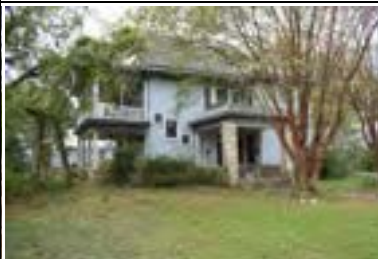
Address: 613 W 32 St (A) Year Built: 1907 HHM ID: 109422 NR Recommendation: Maintain previous listing, Within district
