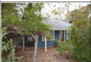
Address: 711 W 35 St (A) Year Built: 1932 HHM ID: 108167 NR Recommendation: Within district
