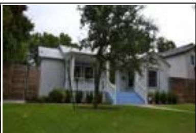
Address: 3207 Beverly Rd Year Built: 1940 HHM ID: 96208 NR Recommendation: Update previous district listing
