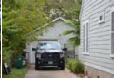
Address: 615 W 35 St (B) Year Built: 1932 HHM ID: 108110 NR Recommendation: Within district
