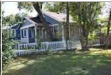
Address: 407 W 37 St Year Built: 1930 HHM ID: 107334 NR Recommendation: Individually eligible, Within district
