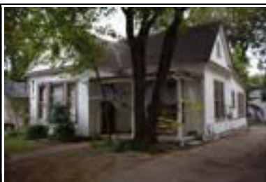
Address: 4513 Avenue B (A) Year Built: 1906 HHM ID: 103627 NR Recommendation: Individually eligible, Within district
