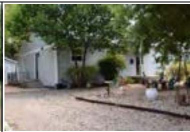
Address: 3209 Bryker Dr (A) Year Built: 1940 HHM ID: 96132 NR Recommendation: Maintain previous district listing
