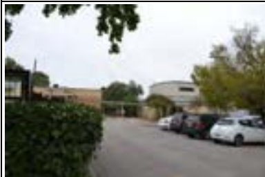
Address: 3309 Kerbey Ln Year Built: 1939 HHM ID: 96694 NR Recommendation: Individually eligible, Add to listed district
