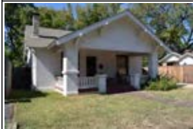
Address: 3310 Jefferson St Year Built: 1920 HHM ID: 98452 NR Recommendation: Maintain previous district listing
