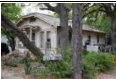
Address: 3404 Grooms St Year Built: 1930 HHM ID: 105400 NR Recommendation: Within district
