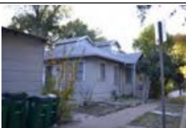
Address: 1107 W 22 St (A) Year Built: 1920 HHM ID: 109898 NR Recommendation: Within district
