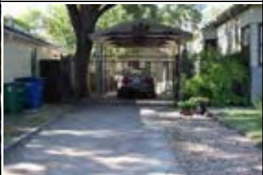
Address: 3102 Kerbey Ln (B) Year Built: 1970 HHM ID: 98642 NR Recommendation: Maintain previous district listing
