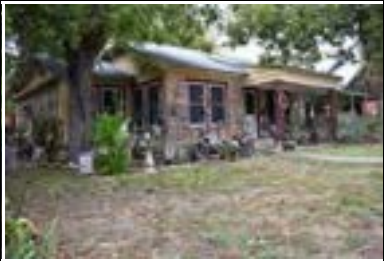
Address: 4600 Avenue H (A) Year Built: 1930 HHM ID: 104171 NR Recommendation: Within district
