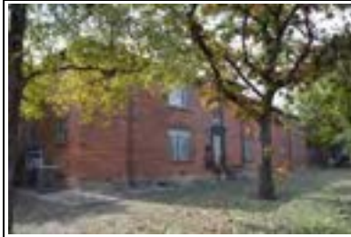
Address: 307 E 33 St (A) Year Built: 1949 HHM ID: 107726 NR Recommendation: Individually eligible, Within district
