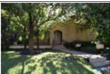
Address: 1521 W 30 St Year Built: 1940 HHM ID: 98570 NR Recommendation: Maintain previous district listing
