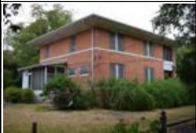
Address: 4600 Caswell Ave (A) Year Built: 1920 HHM ID: 97013 NR Recommendation: Individually eligible, Within district
