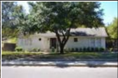
Address: 3112 Kerbey Ln Year Built: 1938 HHM ID: 98485 NR Recommendation: Maintain previous district listing
