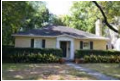
Address: 1511 W 30 St Year Built: 1937 HHM ID: 98919 NR Recommendation: Maintain previous district listing
