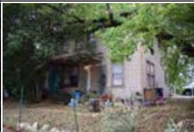
Address: 204 E 30 St (A) Year Built: 1925 HHM ID: 108476 NR Recommendation: Within district
