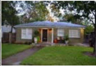
Address: 3305 Glenview Ave Year Built: 1940 HHM ID: 98067 NR Recommendation: Maintain previous district listing
