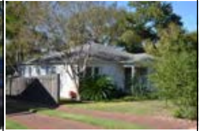
Address: 1717 W 30 St Year Built: 1941 HHM ID: 98286 NR Recommendation: Maintain previous district listing
