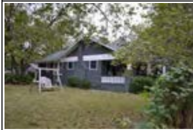
Address: 1114 W 22 1/2 St (A) Year Built: 1935 HHM ID: 109981 NR Recommendation: Within district
