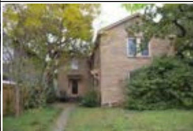
Address: 703 W 35 St (A) Year Built: 1939 HHM ID: 108132 NR Recommendation: Within district
