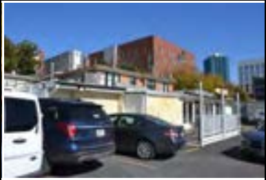
Address: 600 W M L King Jr Blvd Year Built: 1969 HHM ID: 111314 NR Recommendation: Not eligible
