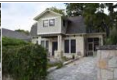
Address: 808 W 32 St Year Built: 1910 HHM ID: 108279 NR Recommendation: Individually eligible, Within district
