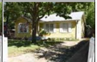
Address: 1702 W 32 St Year Built: 1953 HHM ID: 98352 NR Recommendation: Maintain previous district listing
