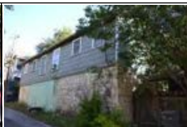
Address: 1104 W M L King Jr Blvd (A) Year Built: 1937 HHM ID: 110953 NR Recommendation: Within district
