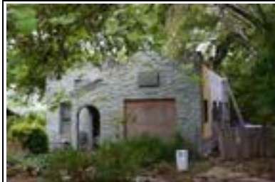
Address: 4702 Rowena St Year Built: 1925 HHM ID: 97921 NR Recommendation: Within district
