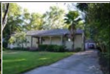
Address: 1505 W 32 St (A) Year Built: 1939 HHM ID: 98716 NR Recommendation: Update previous district listing
