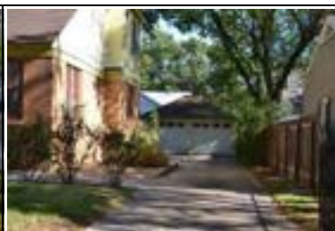
Address: 1502 W 29 St (A) Year Built: 1938 HHM ID: 98838 NR Recommendation: Maintain previous district listing
