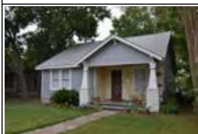
Address: 807 E 45 1/2 St (A) Year Built: 1938 HHM ID: 97137 NR Recommendation: Within district
