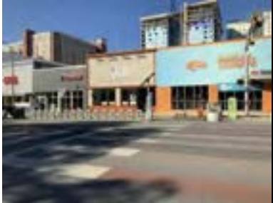
Address: 2232 Guadalupe St (B) Year Built: 1930 HHM ID: 110864 NR Recommendation: Within district
