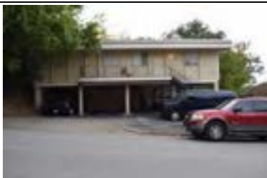
Address: 3115 Owen Ave (A) Year Built: 1965 HHM ID: 108266 NR Recommendation: Within district
