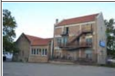
Address: 408 W 23 St Year Built: 1925 HHM ID: 111461 NR Recommendation: Individually eligible
