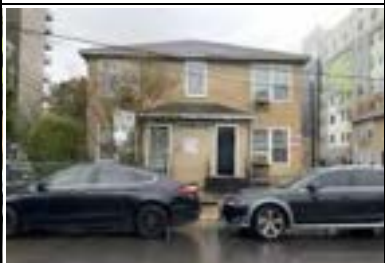
Address: 613 W 24 1/2 St (A) Year Built: 1933 HHM ID: 110682 NR Recommendation: Not eligible
