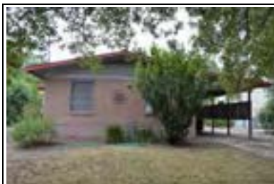
Address: 4808 Red River St Year Built: 1956 HHM ID: 96779 NR Recommendation: Within district
