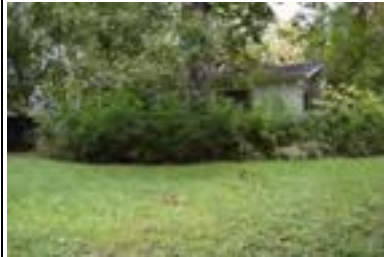
Address: 4521 Avenue D Year Built: 1957 HHM ID: 103946 NR Recommendation: Within district
