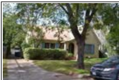
Address: 2842 San Gabriel St (A) Year Built: 1941 HHM ID: 109513 NR Recommendation: Within district
