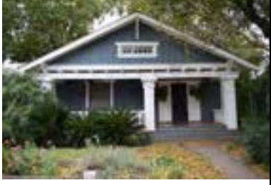
Address: 613 W 31 1/2 St (A) Year Built: 1922 HHM ID: 109188 NR Recommendation: Individually eligible, Within district
