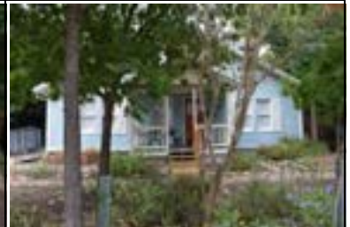
Address: 5008 Caswell Ave Year Built: 1932 HHM ID: 96730 NR Recommendation: Within district
