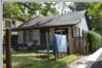
Address: 603 E 49 St (A) Year Built: 1935 HHM ID: 97414 NR Recommendation: Within district
