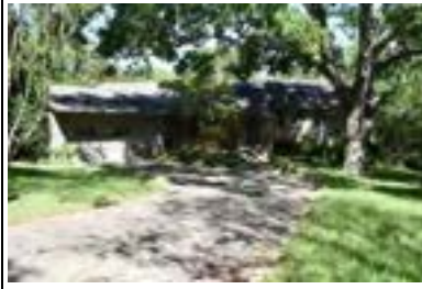
Address: 1304 Belmont Pkwy Year Built: 1960 HHM ID: 99099 NR Recommendation: Add to listed district
