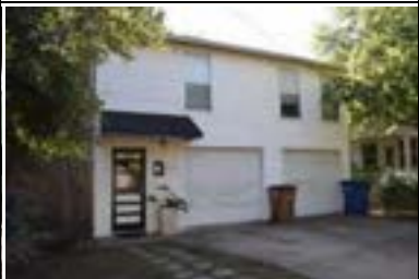
Address: 1410 W 29 St (B) Year Built: 1940 HHM ID: 98852 NR Recommendation: Maintain previous district listing
