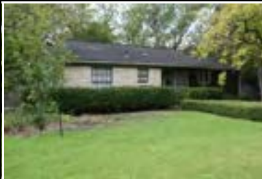
Address: 1901 W 33 St Year Built: 1947 HHM ID: 96000 NR Recommendation: Update previous district listing
