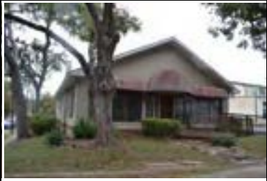
Address: 912 W M L King Jr Blvd Year Built: 1935 HHM ID: 110441 NR Recommendation: Not eligible
