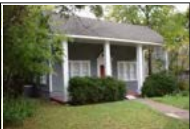
Address: 615 W 31 1/2 St Year Built: 1928 HHM ID: 109193 NR Recommendation: Individually eligible, Within district
