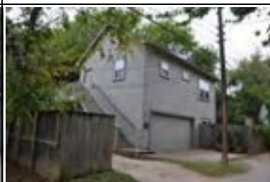
Address: 4515 Avenue G (B) Year Built: 1937 HHM ID: 103085 NR Recommendation: Within district
