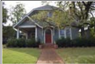
Address: 811 W 31 St (A) Year Built: 1930 HHM ID: 109568 NR Recommendation: Individually eligible, Within district
