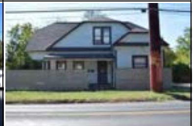
Address: 209 E 38 St Year Built: 1930 HHM ID: 105299 NR Recommendation: Individually eligible, Within district
