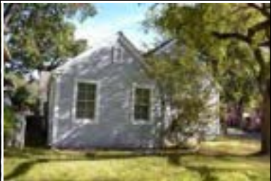
Address: 3500 Tom Green St Year Built: 1938 HHM ID: 105005 NR Recommendation: Within district
