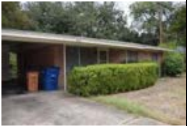
Address: 1700 W 29 St Year Built: 1958 HHM ID: 96530 NR Recommendation: Update previous district listing
