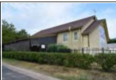
Address: 5002 Caswell Ave Year Built: 1942 HHM ID: 96744 NR Recommendation: Within district
