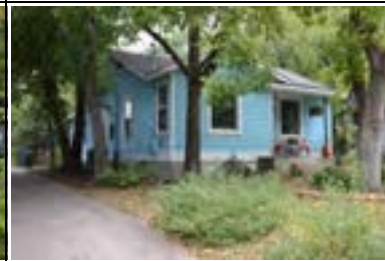
Address: 508 E 49 St (A) Year Built: 1951 HHM ID: 97751 NR Recommendation: Within district
