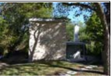
Address: 3215 Churchill Dr Year Built: 1941 HHM ID: 98623 NR Recommendation: Maintain previous listing, Maintain previous district listing
