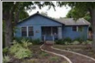
Address: 609 E 50 St (A) Year Built: 1949 HHM ID: 97679 NR Recommendation: Within district
