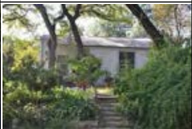
Address: 2834 Shoal Crest Ave Year Built: 1938 HHM ID: 109601 NR Recommendation: Within district
