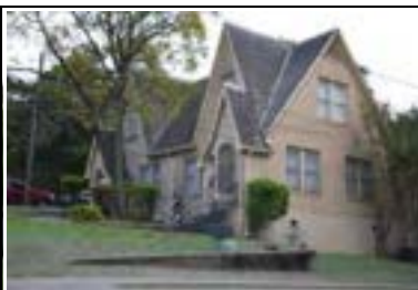
Address: 407 E 32 St Year Built: 1934 HHM ID: 107999 NR Recommendation: Individually eligible, Within district
