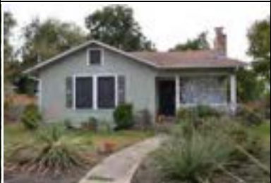
Address: 801 E 48 St (A) Year Built: 1949 HHM ID: 96916 NR Recommendation: Within district
