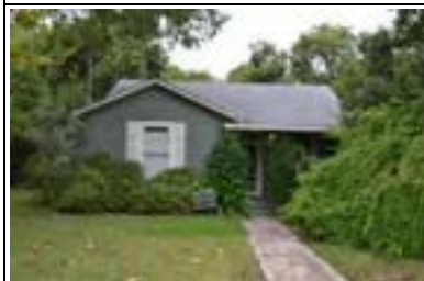
Address: 4708 Rowena St Year Built: 1950 HHM ID: 97905 NR Recommendation: Within district
