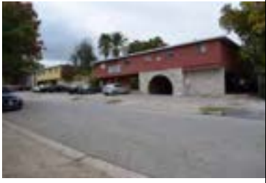
Address: 2907 West Ave Year Built: 1971 HHM ID: 109022 NR Recommendation: Within district
