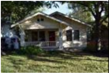
Address: 3011 West Ave Year Built: 1921 HHM ID: 109846 NR Recommendation: Individually eligible, Within district
