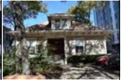
Address: 608 W 22 St Year Built: 1920 HHM ID: 111029 NR Recommendation: Individually eligible
