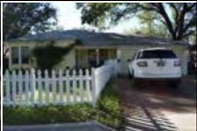
Address: 3100 Kerbey Ln Year Built: 1939 HHM ID: 98646 NR Recommendation: Update previous district listing
