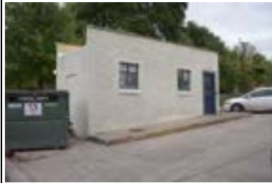
Address: 2900 Rio Grande St (B) Year Built: 1952 HHM ID: 108992 NR Recommendation: Within district
