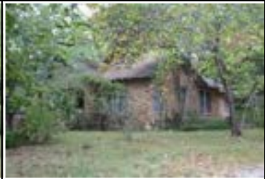
Address: 4612 Red River St (A) Year Built: 1930 HHM ID: 97094 NR Recommendation: Individually eligible, Within district
