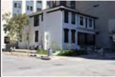
Address: 506 W 22 St Year Built: 1877 HHM ID: 111129 NR Recommendation: Individually eligible
