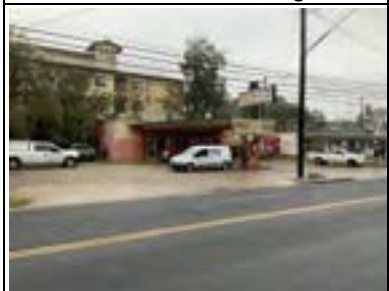
Address: 907 W 24 St Year Built: 1965 HHM ID: 110654 NR Recommendation: Individually eligible
