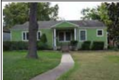
Address: 1907 W 33 St (A) Year Built: 1947 HHM ID: 95973 NR Recommendation: Maintain previous district listing
