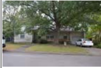
Address: 1907 W 34 St Year Built: 1950 HHM ID: 95918 NR Recommendation: Maintain previous district listing
