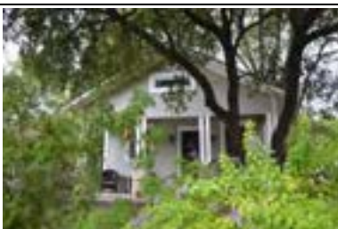
Address: 4714 Avenue H (A) Year Built: 1922 HHM ID: 104403 NR Recommendation: Within district
