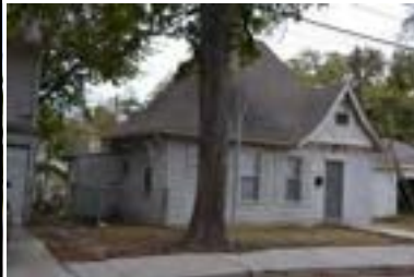
Address: 1100 W 22 St (C) Year Built: 1935 HHM ID: 110137 NR Recommendation: Individually eligible, Within district
