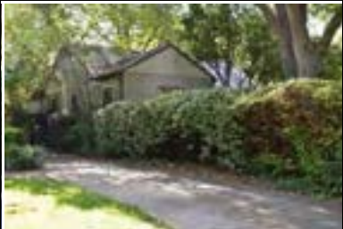
Address: 2905 Glenview Ave (A) Year Built: 1938 HHM ID: 98262 NR Recommendation: Maintain previous district listing
