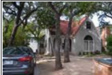
Address: 2830 San Gabriel St Year Built: 1930 HHM ID: 109483 NR Recommendation: Within district
