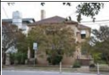
Address: 3305 Speedway Year Built: 1930 HHM ID: 107659 NR Recommendation: Within district
