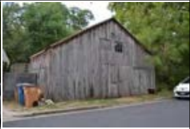
Address: 4529 Avenue G (C) Year Built: 1925 HHM ID: 103053 NR Recommendation: Within district
