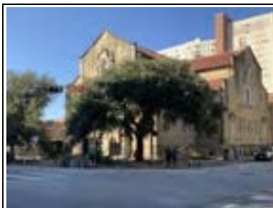
Address: 2130 Guadalupe St Year Built: 1921 HHM ID: 110806 NR Recommendation: Maintain previous listing, Within district
