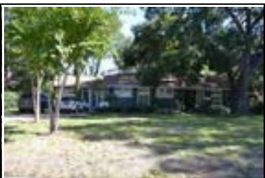
Address: 2907 Oakhurst Ave Year Built: 1951 HHM ID: 99126 NR Recommendation: Add to listed district
