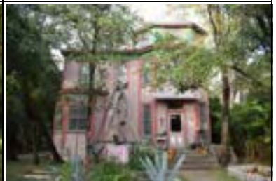
Address: 702 W 32 St Year Built: 1890 HHM ID: 108334 NR Recommendation: Individually eligible, Within district
