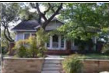
Address: 2838 Shoal Crest Ave Year Built: 1930 HHM ID: 109777 NR Recommendation: Within district
