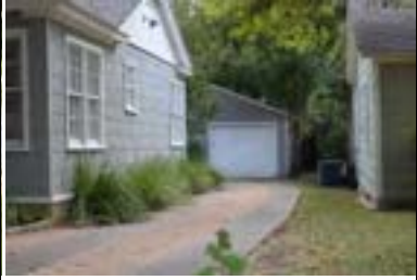
Address: 3303 Oakmont Blvd (B) Year Built: 1948 HHM ID: 96026 NR Recommendation: Maintain previous district listing
