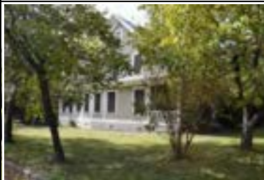
Address: 701 W 32 St (A) Year Built: 1907 HHM ID: 109600 NR Recommendation: Individually eligible, Within district
