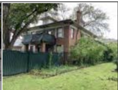
Address: 2402 Rio Grande St Year Built: 1920 HHM ID: 110634 NR Recommendation: Individually eligible
