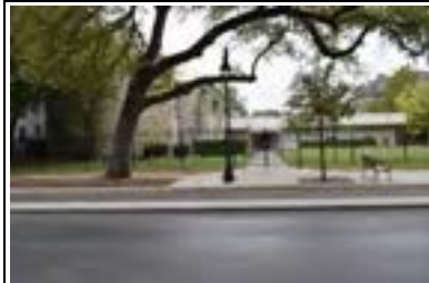
Address: 2614 Rio Grande St Year Built: 1961 HHM ID: 110446 NR Recommendation: Individually eligible
