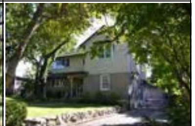
Address: 3101 Beverly Rd Year Built: 1945 HHM ID: 98323 NR Recommendation: Update previous district listing
