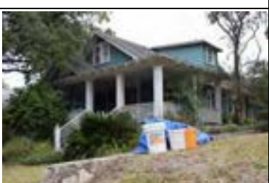
Address: 904 W 30 St Year Built: 1919 HHM ID: 110111 NR Recommendation: Individually eligible, Within district
