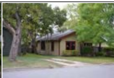
Address: 4703 Avenue G Year Built: 1925 HHM ID: 102991 NR Recommendation: Individually eligible, Within district
