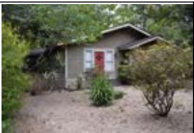
Address: 3212 Oakmont Blvd Year Built: 1948 HHM ID: 96470 NR Recommendation: Update previous district listing
