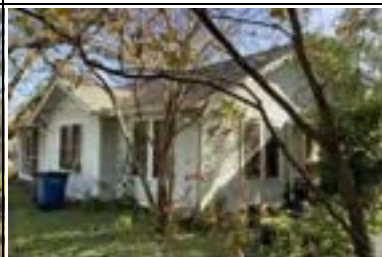
Address: 300 Moore Blvd Year Built: 1929 HHM ID: 107953 NR Recommendation: Individually eligible, Within district
