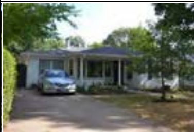
Address: 1802 W 34 St Year Built: 1953 HHM ID: 95883 NR Recommendation: Maintain previous district listing
