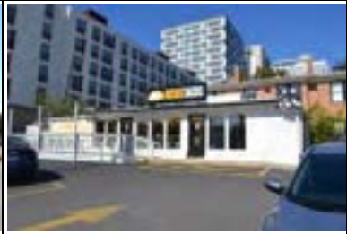
Address: 600 W M L King Jr Blvd Year Built: 1969 HHM ID: 111314 NR Recommendation: Not eligible
