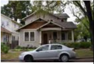
Address: 500 W 43 St (A) Year Built: 1922 HHM ID: 103430 NR Recommendation: Within district
