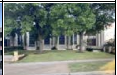
Address: 1909 University Ave (A) Year Built: 1960 HHM ID: 111205 NR Recommendation: Individually eligible
