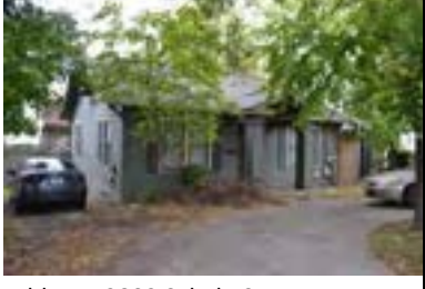
Address: 2802 Salado St Year Built: 1928 HHM ID: 109184 NR Recommendation: Not eligible
