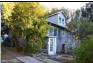
Address: 1107 W 22 St (A) Year Built: 1920 HHM ID: 109898 NR Recommendation: Within district
