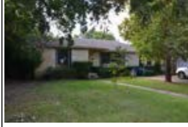
Address: 1911 W 34 St Year Built: 1951 HHM ID: 95934 NR Recommendation: Update previous district listing
