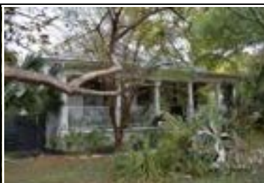
Address: 610 W 32 St Year Built: 1907 HHM ID: 109408 NR Recommendation: Individually eligible, Within district
