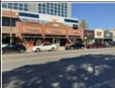
Address: 2326 Guadalupe St (B) Year Built: 1945 HHM ID: 110897 NR Recommendation: Within district
