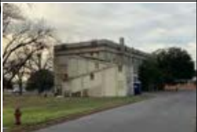
Address: 4110 Guadalupe St (D) Year Built: 1925 HHM ID: 113344 NR Recommendation: Individually eligible, Within district
