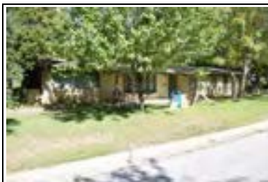
Address: 612 E 48 St Year Built: 1953 HHM ID: 104802 NR Recommendation: Individually eligible, Within district
