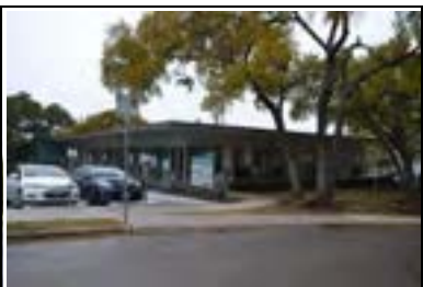
Address: 1201 W 24 St Year Built: 1959 HHM ID: 110536 NR Recommendation: Individually eligible, Within district
