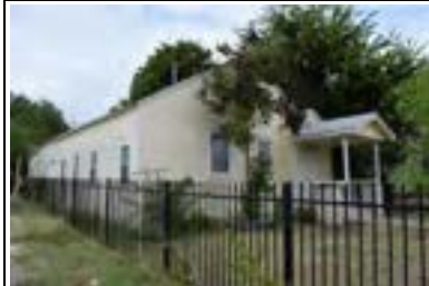
Address: 5006 Caswell Ave Year Built: 1940 HHM ID: 96741 NR Recommendation: Within district
