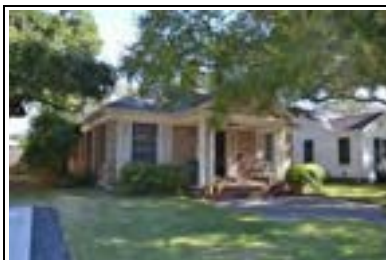
Address: 306 E 35 St Year Built: 1939 HHM ID: 105193 NR Recommendation: Individually eligible, Within district
