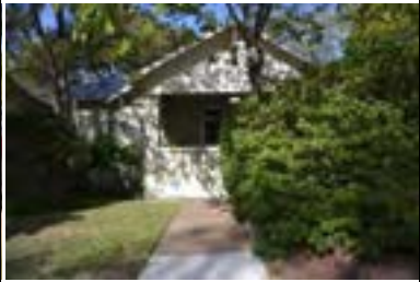
Address: 304 W 34 St (A) Year Built: 1925 HHM ID: 107413 NR Recommendation: Individually eligible, Within district
