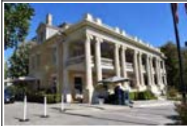
Address: 1900 Rio Grande St Year Built: 1900 HHM ID: 111041 NR Recommendation: Maintain previous listing
