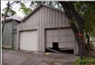
Address: 617 W 32 St (B) Year Built: 1915 HHM ID: 109262 NR Recommendation: Within district
