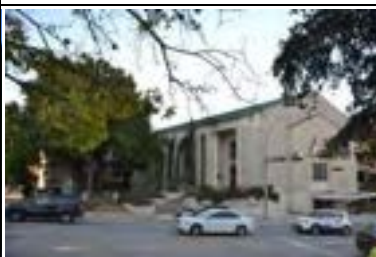
Address: 1909 University Ave (A) Year Built: 1960 HHM ID: 111205 NR Recommendation: Individually eligible
