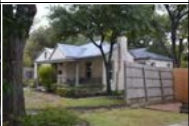
Address: 2308 Longview St Year Built: 1942 HHM ID: 110569 NR Recommendation: Within district
