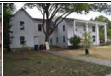
Address: 4612 Caswell Ave Year Built: 1930 HHM ID: 97061 NR Recommendation: Within district
