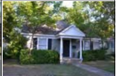
Address: 3313 Glenview Ave (A) Year Built: 1940 HHM ID: 98087 NR Recommendation: Maintain previous district listing
