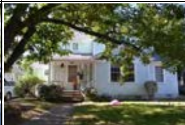
Address: 3204 Kerbey Ln Year Built: 1947 HHM ID: 98574 NR Recommendation: Update previous district listing
