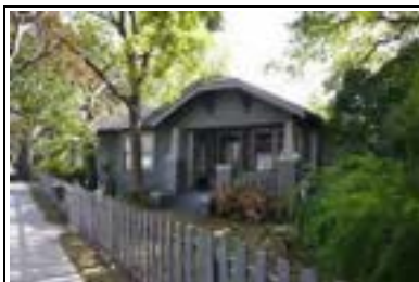
Address: 909 W 29 St Year Built: 1922 HHM ID: 109621 NR Recommendation: Individually eligible, Within district
