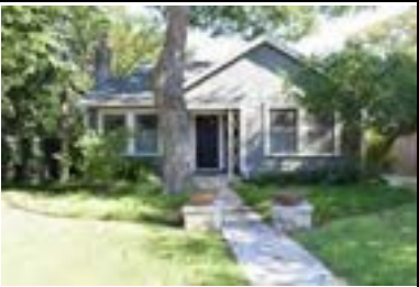
Address: 3003 Kerbey Ln Year Built: 1941 HHM ID: 98577 NR Recommendation: Maintain previous district listing
