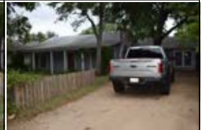
Address: 3210 Oakmont Blvd Year Built: 1947 HHM ID: 96477 NR Recommendation: Update previous district listing
