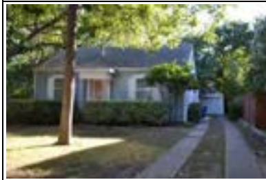
Address: 1513 W 32 St (A) Year Built: 1938 HHM ID: 98704 NR Recommendation: Maintain previous district listing
