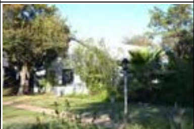
Address: 1208 W 22 St (A) Year Built: 1927 HHM ID: 109845 NR Recommendation: Individually eligible, Within district
