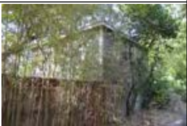
Address: 2839 Shoal Crest Ave (B) Year Built: 1932 HHM ID: 109747 NR Recommendation: Within district
