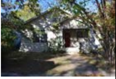
Address: 706 W 30 St (A) Year Built: 1928 HHM ID: 109811 NR Recommendation: Individually eligible, Within district
