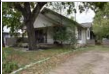
Address: 704 W 35 St Year Built: 1925 HHM ID: 108129 NR Recommendation: Individually eligible, Within district
