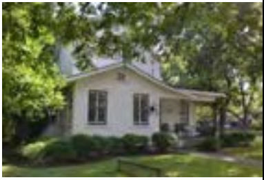
Address: 3301 Glenview Ave (A) Year Built: 1938 HHM ID: 98040 NR Recommendation: Update previous district listing
