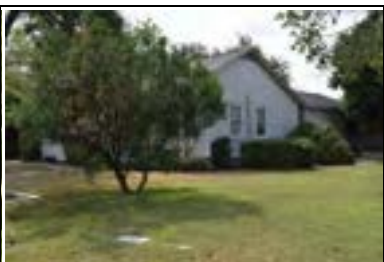
Address: 1903 W 33 St (A) Year Built: 1938 HHM ID: 95992 NR Recommendation: Maintain previous district listing
