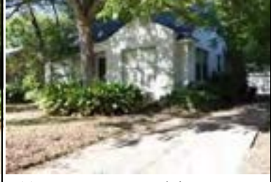
Address: 1518 W 31 St (A) Year Built: 1939 HHM ID: 98612 NR Recommendation: Maintain previous district listing
