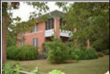
Address: 4600 Caswell Ave (A) Year Built: 1920 HHM ID: 97013 NR Recommendation: Individually eligible, Within district
