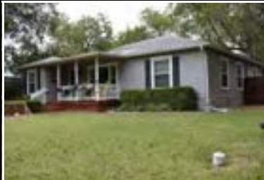
Address: 3105 Funston St Year Built: 1949 HHM ID: 96360 NR Recommendation: Update previous district listing
