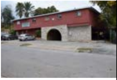
Address: 2907 West Ave Year Built: 1971 HHM ID: 109022 NR Recommendation: Within district
