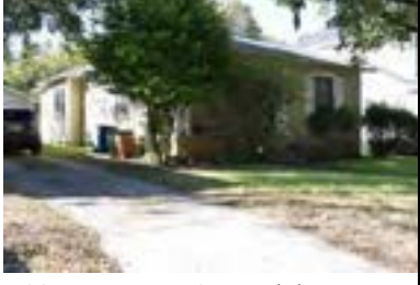
Address: 3302 Kerbey Ln (A) Year Built: 1941 HHM ID: 98662 NR Recommendation: Maintain previous district listing
