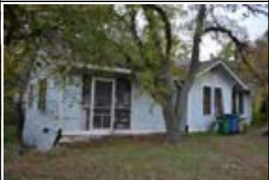
Address: 300 Moore Blvd Year Built: 1929 HHM ID: 107953 NR Recommendation: Individually eligible, Within district
