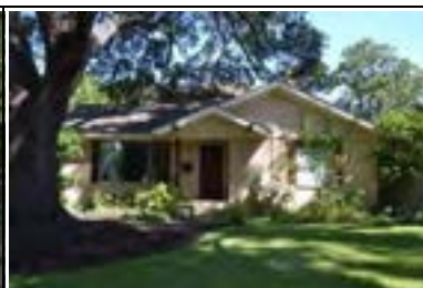
Address: 1704 W 31 St Year Built: 1950 HHM ID: 98355 NR Recommendation: Maintain previous district listing
