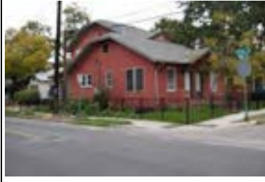
Address: 2900 West Ave Year Built: 1932 HHM ID: 109006 NR Recommendation: Within district
