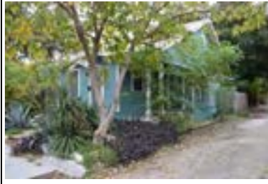
Address: 2904 West Ave Year Built: 1930 HHM ID: 109019 NR Recommendation: Within district
