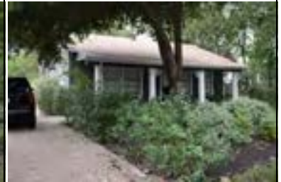
Address: 4612 Avenue D Year Built: 1948 HHM ID: 103848 NR Recommendation: Within district
