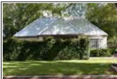
Address: 1804 W 34 St Year Built: 1965 HHM ID: 95887 NR Recommendation: Maintain previous district listing
