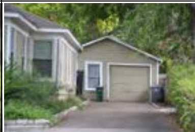
Address: 1906 W 33 St (B) Year Built: 1947 HHM ID: 95978 NR Recommendation: Maintain previous district listing
