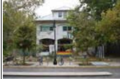
Address: 2610 Rio Grande St Year Built: 1930 HHM ID: 110450 NR Recommendation: Not eligible
