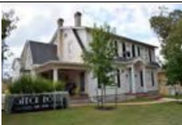
Address: 305 E 34 St Year Built: 1921 HHM ID: 107679 NR Recommendation: Individually eligible, Within district
