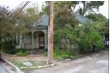
Address: 506 W 42 St Year Built: 1907 HHM ID: 104348 NR Recommendation: Individually eligible, Within district
