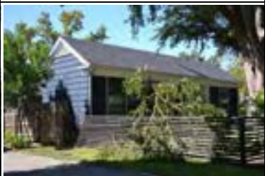
Address: 1707 W 31 St Year Built: 1947 HHM ID: 98351 NR Recommendation: Update previous district listing
