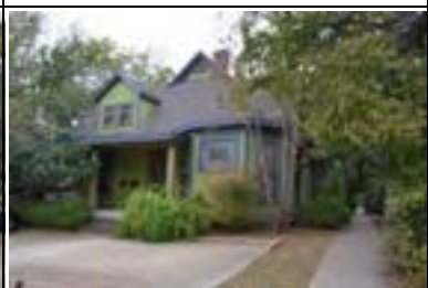
Address: 2110 San Gabriel St (A) Year Built: 1900 HHM ID: 110474 NR Recommendation: Not eligible
