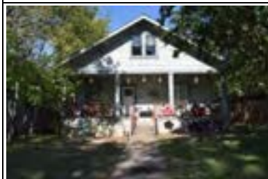
Address: 406 W 37 St Year Built: 1925 HHM ID: 107345 NR Recommendation: Individually eligible, Within district
