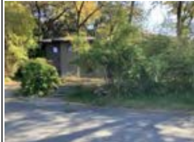
Address: 2301 Shoal Creek Blvd Year Built: 1940 HHM ID: 111357 NR Recommendation: Within district
