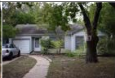
Address: 4911 Duval St (A) Year Built: 1946 HHM ID: 97582 NR Recommendation: Within district
