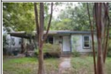
Address: 4511 Avenue D Year Built: 1955 HHM ID: 103935 NR Recommendation: Within district
