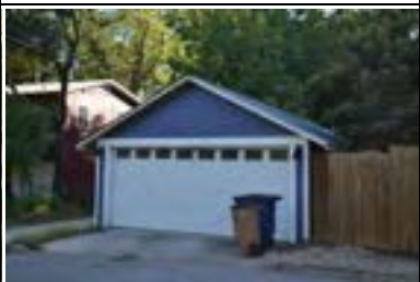
Address: 4717 Avenue G (B) Year Built: 1930 HHM ID: 102904 NR Recommendation: Within district
