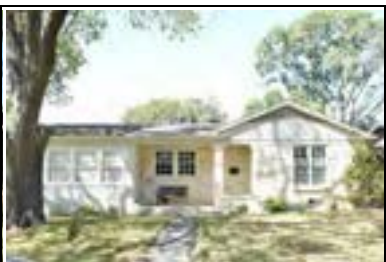
Address: 3004 Bryker Dr Year Built: 1941 HHM ID: 98422 NR Recommendation: Maintain previous district listing
