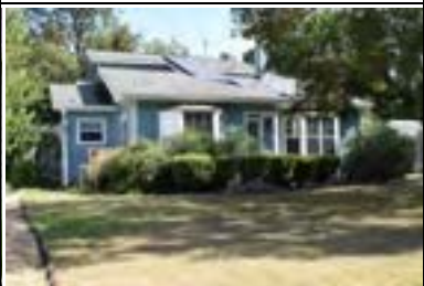
Address: 3207 Bryker Dr Year Built: 1940 HHM ID: 96147 NR Recommendation: Maintain previous district listing
