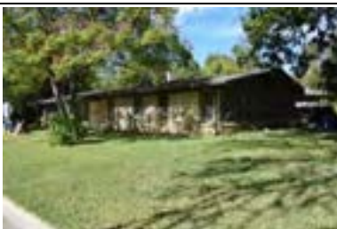
Address: 612 E 48 St Year Built: 1953 HHM ID: 104802 NR Recommendation: Individually eligible, Within district
