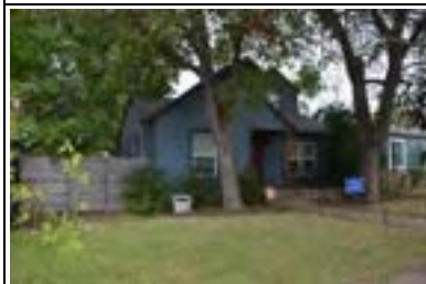
Address: 4508 Red River St Year Built: 1939 HHM ID: 97239 NR Recommendation: Within district
