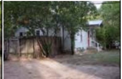
Address: 706 W 32 St (B) Year Built: 1935 HHM ID: 108319 NR Recommendation: Within district
