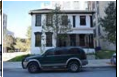
Address: 506 W 22 St Year Built: 1877 HHM ID: 111129 NR Recommendation: Individually eligible
