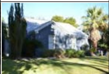
Address: 1506 W 32 St (A) Year Built: 1938 HHM ID: 98732 NR Recommendation: Maintain previous district listing
