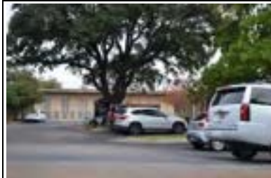
Address: 100 E 27 St (D) Year Built: 1961 HHM ID: 108791 NR Recommendation: Individually eligible, Within district
