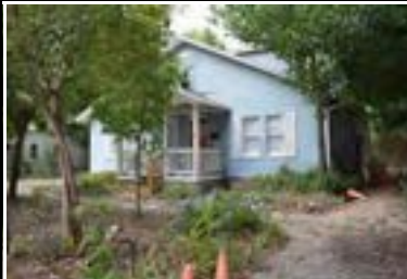
Address: 5008 Caswell Ave Year Built: 1932 HHM ID: 96730 NR Recommendation: Within district
