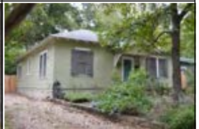
Address: 4528 Avenue D Year Built: 1934 HHM ID: 103809 NR Recommendation: Within district
