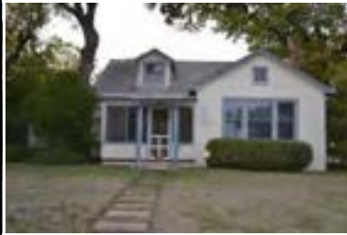
Address: 3114 West Ave Year Built: 1922 HHM ID: 108311 NR Recommendation: Within district
