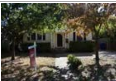
Address: 1519 W 31 St (A) Year Built: 1938 HHM ID: 98601 NR Recommendation: Maintain previous district listing
