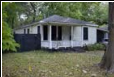
Address: 4527 Avenue D Year Built: 1941 HHM ID: 103924 NR Recommendation: Within district
