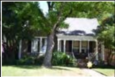
Address: 1514 W 31 St Year Built: 1939 HHM ID: 98993 NR Recommendation: Maintain previous district listing
