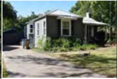
Address: 1515 W 31 St Year Built: 1938 HHM ID: 98991 NR Recommendation: Maintain previous district listing
