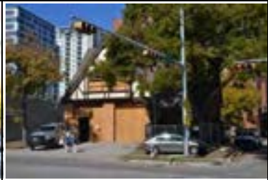
Address: 506 W M L King Jr Blvd Year Built: 1932 HHM ID: 111316 NR Recommendation: Individually eligible
