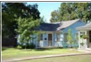
Address: 1702 W 33 St Year Built: 1945 HHM ID: 98444 NR Recommendation: Maintain previous district listing
