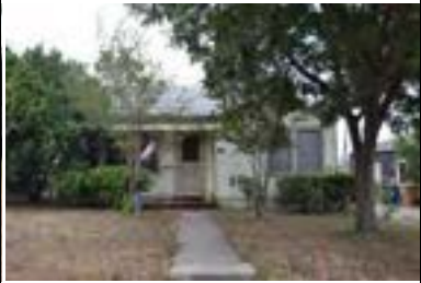
Address: 1702 W 34 St Year Built: 1946 HHM ID: 95860 NR Recommendation: Update previous district listing
