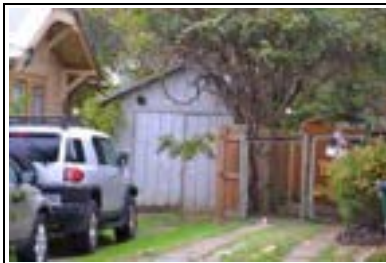
Address: 2832 Pearl St (B) Year Built: 1923 HHM ID: 109321 NR Recommendation: Within district
