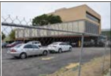
Address: 1213 W 34 St Year Built: 1965 HHM ID: 96679 NR Recommendation: Individually eligible
