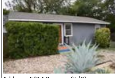
Address: 5014 Rowena St (B) Year Built: 1950 HHM ID: 97832 NR Recommendation: Within district
