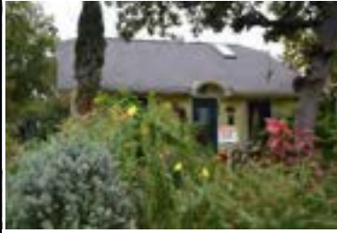
Address: 617 W 35 St (A) Year Built: 1928 HHM ID: 108126 NR Recommendation: Within district
