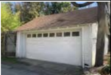
Address: 3006 Fruth St (B) Year Built: 1936 HHM ID: 113289 NR Recommendation: Within district
