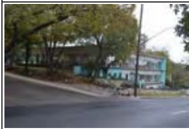
Address: 1201 W 24 St Year Built: 1959 HHM ID: 110536 NR Recommendation: Individually eligible, Within district
