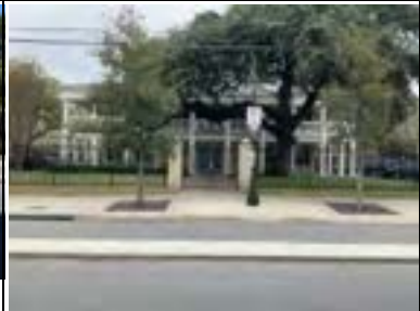
Address: 2508 Rio Grande St Year Built: 1964 HHM ID: 110281 NR Recommendation: Individually eligible
