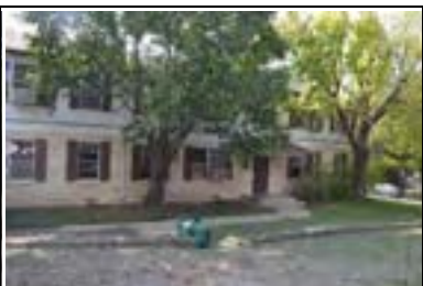
Address: 301 A E 33 St Year Built: 1949 HHM ID: 107727 NR Recommendation: Within district
