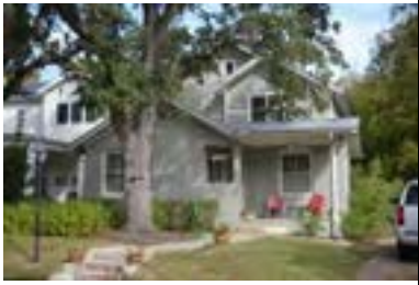
Address: 1504 W 31 St (B) Year Built: 1940 HHM ID: 98967 NR Recommendation: Maintain previous district listing
