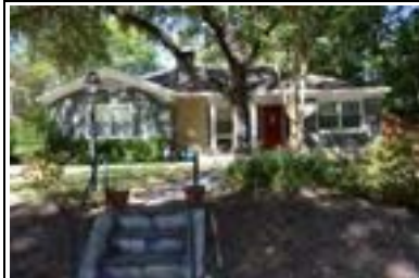
Address: 3104 Beverly Rd Year Built: 1948 HHM ID: 98343 NR Recommendation: Maintain previous district listing
