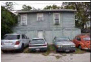
Address: 2910 Fruth St (B) Year Built: 1930 HHM ID: 108555 NR Recommendation: Not eligible
