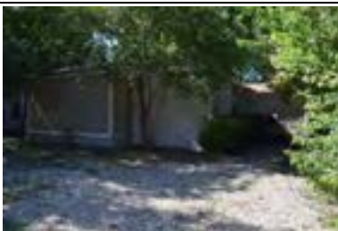
Address: 3306 Jefferson St Year Built: 1955 HHM ID: 98448 NR Recommendation: Maintain previous district listing
