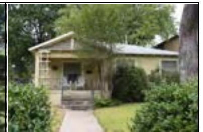
Address: 5000 Duval St (A) Year Built: 1935 HHM ID: 97823 NR Recommendation: Within district
