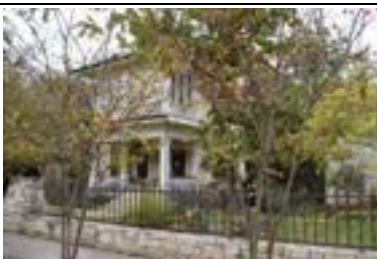
Address: 609 W 33 St (A) Year Built: 1910 HHM ID: 109369 NR Recommendation: Individually eligible, Within district
