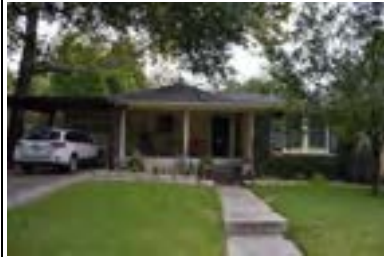
Address: 3205 Oakmont Blvd Year Built: 1949 HHM ID: 96460 NR Recommendation: Maintain previous district listing
