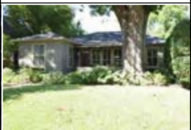
Address: 3102 Bryker Dr Year Built: 1941 HHM ID: 98407 NR Recommendation: Update previous district listing
