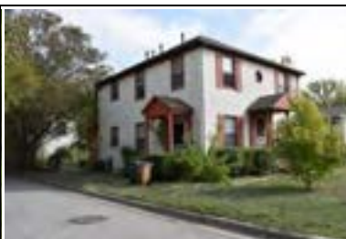
Address: 410 W 34 St (A) Year Built: 1937 HHM ID: 107570 NR Recommendation: Within district
