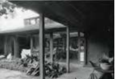
Address: 1901 Cliff St Year Built: 1955 HHM ID: 110693 NR Recommendation: Maintain previous listing, Within district
