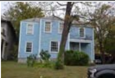
Address: 2307 Longview St Year Built: 1940 HHM ID: 110554 NR Recommendation: Within district
