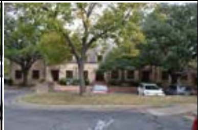
Address: 100 E 27 St (E) Year Built: 1945 HHM ID: 108786 NR Recommendation: Within district
