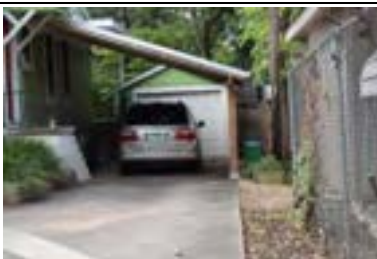
Address: 1907 W 33 St (B) Year Built: 1947 HHM ID: 95981 NR Recommendation: Maintain previous district listing
