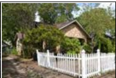
Address: 4520 Red River St Year Built: 1938 HHM ID: 97303 NR Recommendation: Individually eligible, Within district
