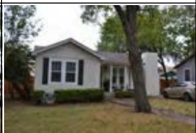
Address: 3202 Funston St Year Built: 1947 HHM ID: 96343 NR Recommendation: Update previous district listing
