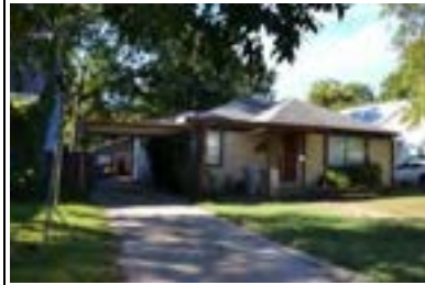
Address: 4704 Evans Ave Year Built: 1946 HHM ID: 104923 NR Recommendation: Within district
