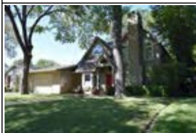
Address: 3100 Bryker Dr Year Built: 1958 HHM ID: 98411 NR Recommendation: Maintain previous district listing
