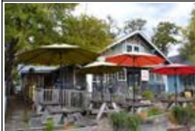
Address: 616 W 34 St Year Built: 1922 HHM ID: 108224 NR Recommendation: Individually eligible, Within district
