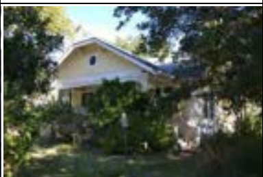
Address: 310 E 34 St Year Built: 1922 HHM ID: 105072 NR Recommendation: Individually eligible, Within district
