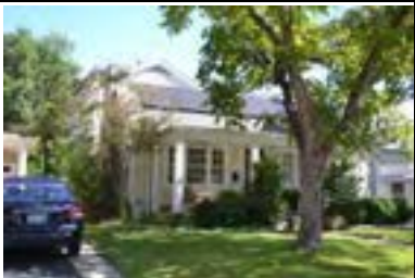
Address: 1506 W 31 St Year Built: 1939 HHM ID: 98951 NR Recommendation: Maintain previous district listing
