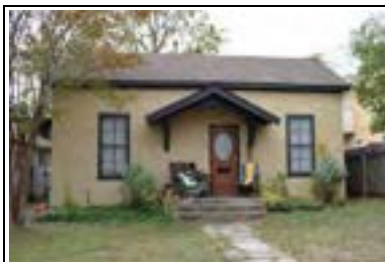
Address: 613 W 37 St (C) Year Built: 1928 HHM ID: 108036 NR Recommendation: Within district
