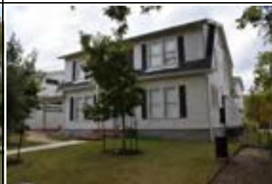
Address: 305 E 34 St Year Built: 1921 HHM ID: 107679 NR Recommendation: Individually eligible, Within district
