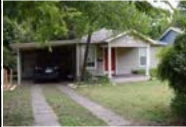
Address: 4609 Avenue D Year Built: 1930 HHM ID: 103864 NR Recommendation: Within district
