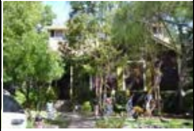
Address: 1516 W 31 St Year Built: 1939 HHM ID: 98994 NR Recommendation: Update previous district listing
