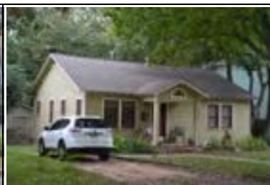
Address: 4527 Avenue C (B) Year Built: 1947 HHM ID: 103757 NR Recommendation: Within district
