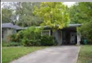
Address: 4530 Avenue D Year Built: 1952 HHM ID: 103808 NR Recommendation: Within district
