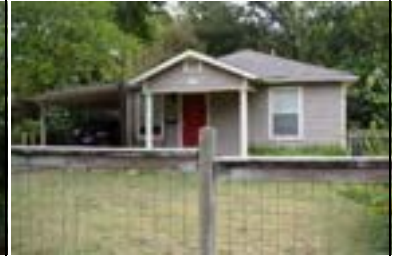
Address: 4609 Avenue D Year Built: 1930 HHM ID: 103864 NR Recommendation: Within district
