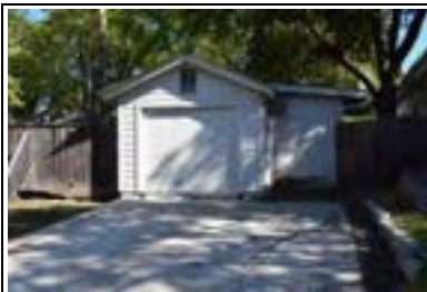
Address: 3000 Beverly Rd (B) Year Built: 1947 HHM ID: 98309 NR Recommendation: Maintain previous district listing
