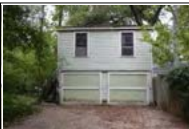
Address: 4529 Avenue D (B) Year Built: 1941 HHM ID: 103913 NR Recommendation: Within district
