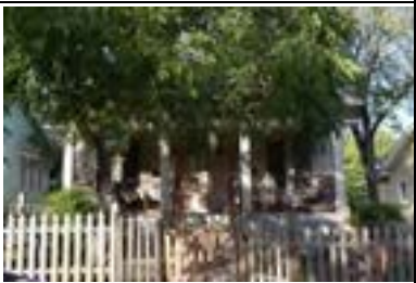
Address: 204 E 34 St (A) Year Built: 1922 HHM ID: 107448 NR Recommendation: Individually eligible, Within district
