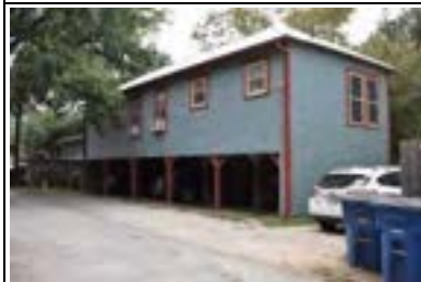
Address: 4413 Avenue A (C) Year Built: 1939 HHM ID: 103339 NR Recommendation: Within district
