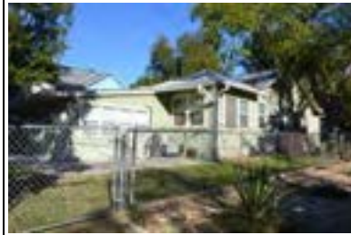
Address: 4700 Evans Ave (A) Year Built: 1940 HHM ID: 104960 NR Recommendation: Within district
