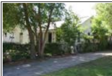
Address: 3004 Kerbey Ln Year Built: 1939 HHM ID: 98497 NR Recommendation: Maintain previous district listing
