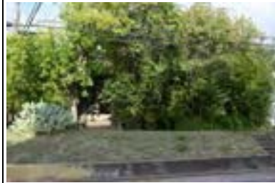
Address: 100 E 30 St (A) Year Built: 1935 HHM ID: 107893 NR Recommendation: Individually eligible, Within district
