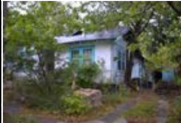
Address: 2835 Pearl St (B) Year Built: 1930 HHM ID: 109332 NR Recommendation: Within district
