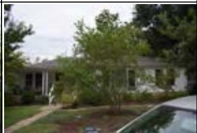
Address: 5000 Evans Ave (A) Year Built: 1947 HHM ID: 97640 NR Recommendation: Within district
