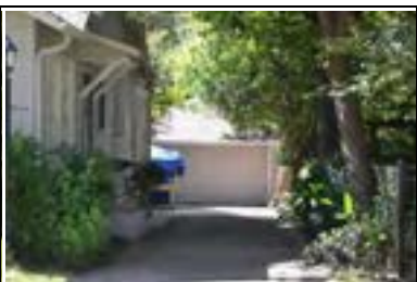
Address: 1703 W 31 St (A) Year Built: 1940 HHM ID: 98349 NR Recommendation: Maintain previous district listing
