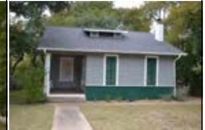
Address: 1910 David St Year Built: 1925 HHM ID: 110310 NR Recommendation: Individually eligible, Within district
