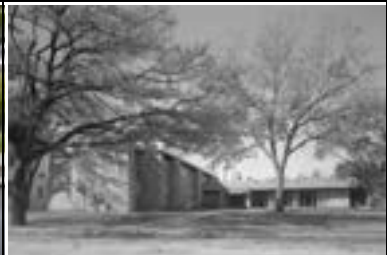
Address: 2614 Rio Grande St Year Built: 1961 HHM ID: 110446 NR Recommendation: Individually eligible
