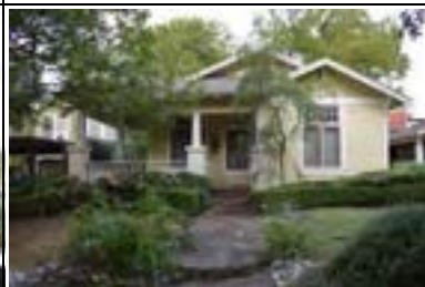
Address: 4714 Avenue G Year Built: 1925 HHM ID: 102953 NR Recommendation: Individually eligible, Within district
