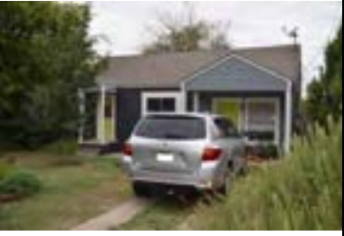
Address: 5014 Rowena St (A) Year Built: 1946 HHM ID: 97835 NR Recommendation: Within district
