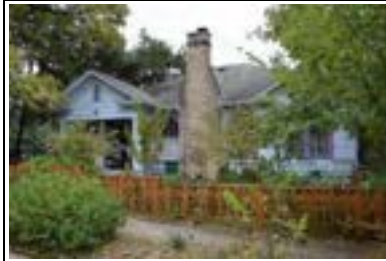
Address: 901 W 30 St (A) Year Built: 1924 HHM ID: 110163 NR Recommendation: Individually eligible, Within district
