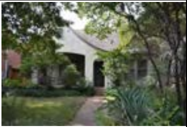
Address: 2834 San Gabriel St Year Built: 1932 HHM ID: 109459 NR Recommendation: Within district
