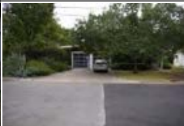
Address: 4607 Caswell Ave Year Built: 1961 HHM ID: 97043 NR Recommendation: Within district
