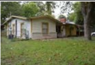
Address: 4600 Avenue D Year Built: 1952 HHM ID: 103831 NR Recommendation: Within district
