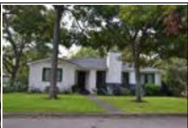
Address: 1901 W 34 St Year Built: 1949 HHM ID: 95897 NR Recommendation: Maintain previous district listing
