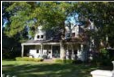
Address: 3102 Glenview Ave Year Built: 1938 HHM ID: 98191 NR Recommendation: Maintain previous district listing
