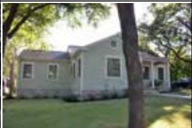
Address: 1517 W 32 St Year Built: 1939 HHM ID: 98669 NR Recommendation: Maintain previous district listing
