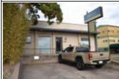
Address: 700 W 34 St (A) Year Built: 1955 HHM ID: 108207 NR Recommendation: Within district
