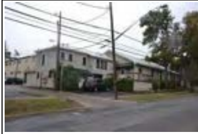
Address: 912 W M L King Jr Blvd Year Built: 1935 HHM ID: 110441 NR Recommendation: Not eligible
