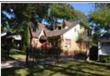
Address: 1502 W 29 St (A) Year Built: 1938 HHM ID: 98838 NR Recommendation: Maintain previous district listing
