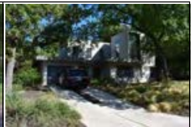
Address: 1708 W 30 St Year Built: 1947 HHM ID: 98287 NR Recommendation: Update previous district listing
