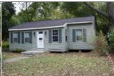
Address: 4604 Avenue D Year Built: 1942 HHM ID: 103835 NR Recommendation: Within district
