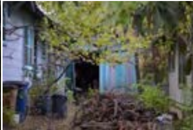
Address: 2835 Pearl St (B) Year Built: 1930 HHM ID: 109332 NR Recommendation: Within district
