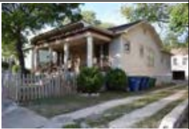
Address: 204 E 34 St (A) Year Built: 1922 HHM ID: 107448 NR Recommendation: Individually eligible, Within district
