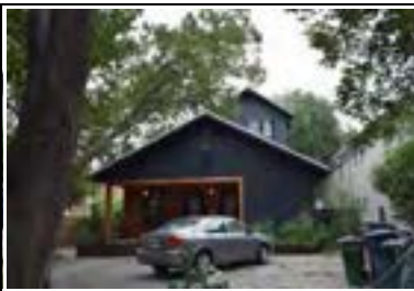
Address: 4408 Avenue A Year Built: 1925 HHM ID: 103360 NR Recommendation: Within district
