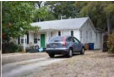
Address: 1702 W 29 St (A) Year Built: 1939 HHM ID: 96539 NR Recommendation: Maintain previous district listing
