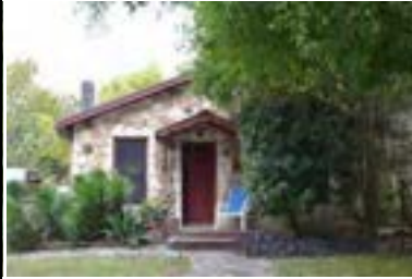
Address: 4520 Avenue D Year Built: 1935 HHM ID: 103812 NR Recommendation: Within district
