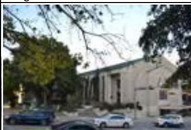
Address: 1909 University Ave (A) Year Built: 1960 HHM ID: 111205 NR Recommendation: Individually eligible
