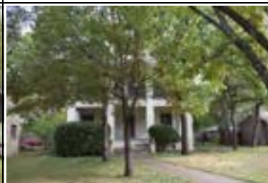
Address: 614 W 32 St Year Built: 1901 HHM ID: 109437 NR Recommendation: Individually eligible, Within district
