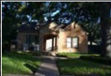
Address: 3207 Glenview Ave (A) Year Built: 1939 HHM ID: 98109 NR Recommendation: Maintain previous district listing
