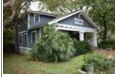
Address: 613 W 31 1/2 St (A) Year Built: 1922 HHM ID: 109188 NR Recommendation: Individually eligible, Within district
