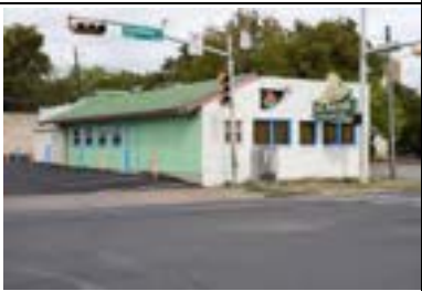
Address: 2934 Guadalupe St (A) Year Built: 1938 HHM ID: 108717 NR Recommendation: Within district
