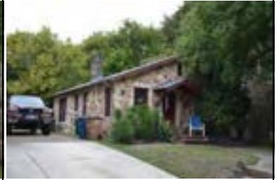
Address: 4520 Avenue D Year Built: 1935 HHM ID: 103812 NR Recommendation: Within district
