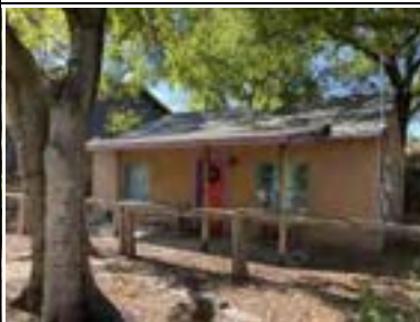
Address: 5002 Avenue F (A) Year Built: 1947 HHM ID: 102795 NR Recommendation: Within district
