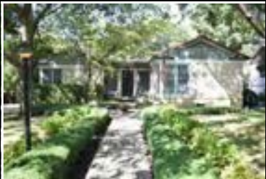
Address: 3006 Beverly Rd Year Built: 1941 HHM ID: 98321 NR Recommendation: Maintain previous district listing
