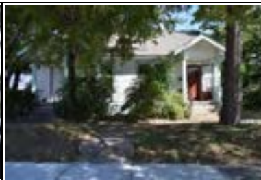
Address: 104 E 35 St (A) Year Built: 1925 HHM ID: 105226 NR Recommendation: Individually eligible, Within district
