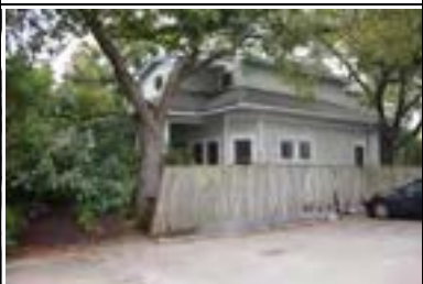
Address: 4304 Avenue A Year Built: 1895 HHM ID: 103415 NR Recommendation: Within district
