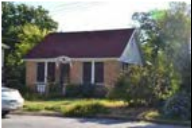
Address: 3407 Tom Green St Year Built: 1933 HHM ID: 105101 NR Recommendation: Within district
