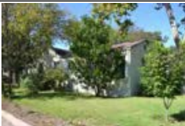
Address: 3200 Kerbey Ln Year Built: 1939 HHM ID: 98484 NR Recommendation: Update previous district listing
