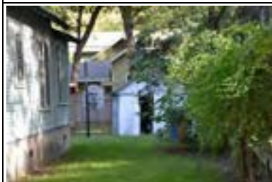
Address: 4603 Avenue B (B) Year Built: 1925 HHM ID: 103549 NR Recommendation: Within district
