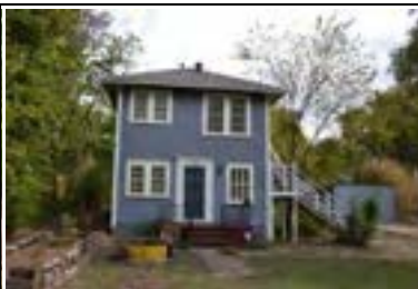
Address: 3205 Tom Green St (A) Year Built: 1935 HHM ID: 107799 NR Recommendation: Within district
