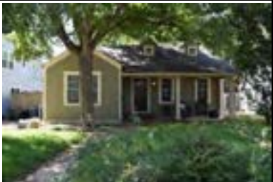
Address: 1511 W 31 St Year Built: 1939 HHM ID: 98971 NR Recommendation: Maintain previous district listing
