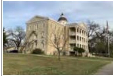
Address: 4110 Guadalupe St (A) Year Built: 1857 HHM ID: 113311 NR Recommendation: Maintain previous listing, Within district
