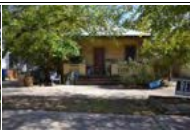
Address: 3411 Cedar St (A) Year Built: 1932 HHM ID: 107016 NR Recommendation: Individually eligible, Within district
