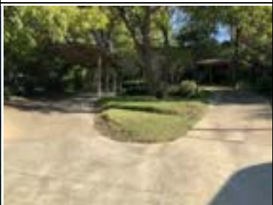
Address: 2311 Shoal Creek Blvd Year Built: 1949 HHM ID: 111373 NR Recommendation: Individually eligible, Within district
