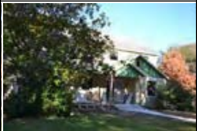
Address: 3104 Glenview Ave Year Built: 1939 HHM ID: 98185 NR Recommendation: Maintain previous district listing
