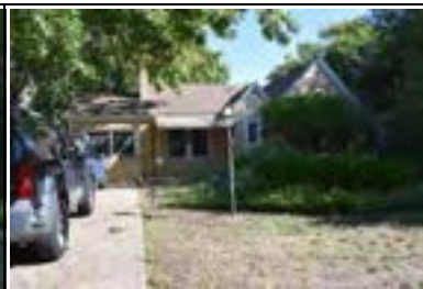
Address: 1510 W 30 St Year Built: 1937 HHM ID: 98908 NR Recommendation: Update previous district listing
