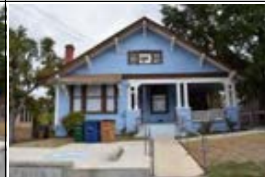
Address: 604 W 35 St Year Built: 1914 HHM ID: 108060 NR Recommendation: Individually eligible, Within district
