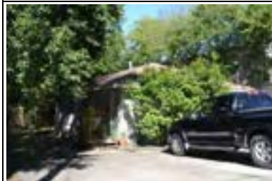
Address: 5002 Rowena St Year Built: 1950 HHM ID: 102732 NR Recommendation: Within district
