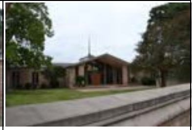
Address: 100 E 27 St (A) Year Built: 1961 HHM ID: 108757 NR Recommendation: Individually eligible, Within district
