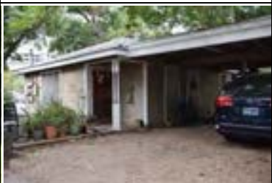
Address: 4600 Avenue B (B) Year Built: 1935 HHM ID: 103513 NR Recommendation: Within district
