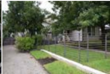
Address: 3208 Oakmont Blvd Year Built: 1946 HHM ID: 96481 NR Recommendation: Maintain previous district listing
