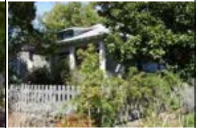
Address: 204 E 35 St Year Built: 1917 HHM ID: 105281 NR Recommendation: Individually eligible, Within district
