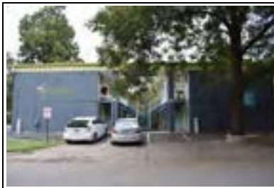
Address: 4400 Avenue A Year Built: 1972 HHM ID: 103364 NR Recommendation: Within district
