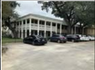
Address: 2508 Rio Grande St Year Built: 1964 HHM ID: 110281 NR Recommendation: Individually eligible
