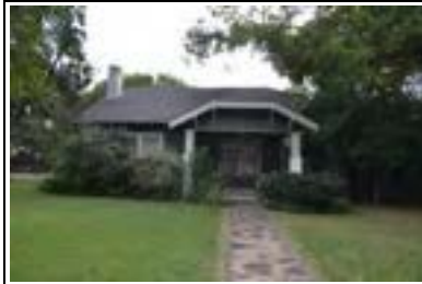
Address: 4529 Avenue G (A) Year Built: 1922 HHM ID: 103045 NR Recommendation: Individually eligible, Within district
