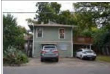
Address: 801 E 48 St (B) Year Built: 1960 HHM ID: 96915 NR Recommendation: Within district
