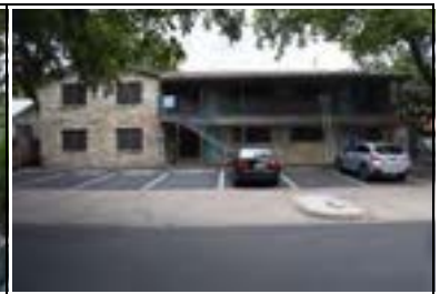
Address: 4409 Avenue A Year Built: 1967 HHM ID: 103353 NR Recommendation: Within district
