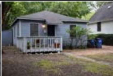
Address: 4525 Avenue D (A) Year Built: 1949 HHM ID: 103938 NR Recommendation: Within district
