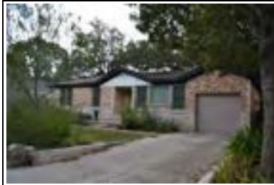
Address: 1903 W 34 St Year Built: 1949 HHM ID: 95904 NR Recommendation: Maintain previous district listing
