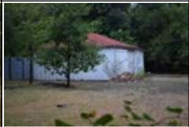
Address: 4600 Caswell Ave Year Built: 1920 HHM ID: 97014 NR Recommendation: Within district
