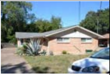
Address: 4906 Rowena St Year Built: 1963 HHM ID: 102754 NR Recommendation: Within district
