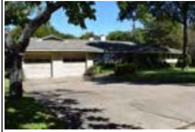
Address: 1302 Belmont Pkwy Year Built: 1960 HHM ID: 99107 NR Recommendation: Add to listed district
