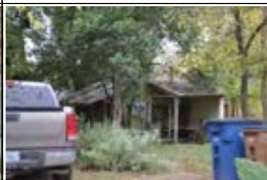
Address: 303 Moore Blvd Year Built: 1933 HHM ID: 108523 NR Recommendation: Within district
