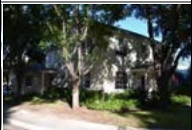
Address: 1508 W 32 St Year Built: 1939 HHM ID: 98723 NR Recommendation: Update previous district listing
