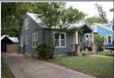
Address: 4508 Avenue B (A) Year Built: 1936 HHM ID: 103678 NR Recommendation: Within district
