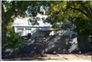
Address: 3213 Kerbey Ln Year Built: 1941 HHM ID: 98488 NR Recommendation: Update previous district listing
