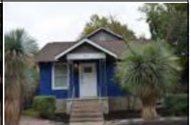
Address: 2913 Rio Grande St Year Built: 1935 HHM ID: 108902 NR Recommendation: Within district
