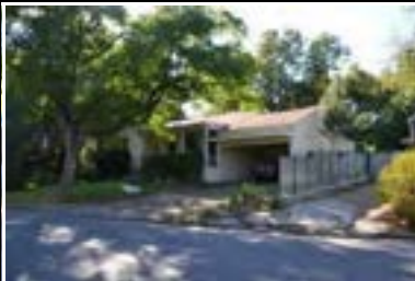
Address: 3204 Churchill Dr Year Built: 1941 HHM ID: 98639 NR Recommendation: Maintain previous district listing
