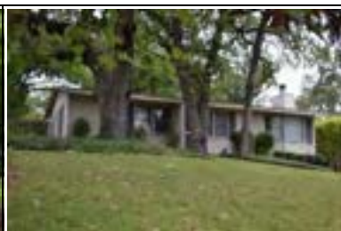
Address: 3007 Oakmont Blvd Year Built: 1955 HHM ID: 96426 NR Recommendation: Update previous district listing
