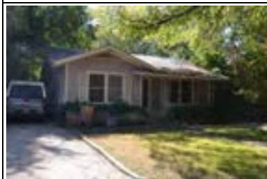
Address: 1703 W 33 St Year Built: 1952 HHM ID: 98445 NR Recommendation: Update previous district listing
