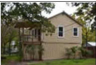
Address: 705 W 35 St (B) Year Built: 1931 HHM ID: 108153 NR Recommendation: Within district
