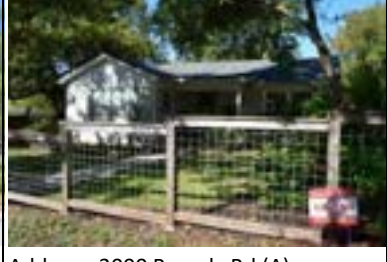
Address: 3000 Beverly Rd (A) Year Built: 1947 HHM ID: 98294 NR Recommendation: Maintain previous district listing
