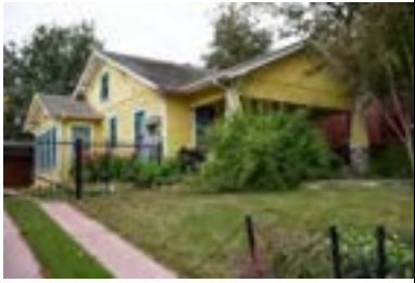
Address: 615 W 30 St Year Built: 1930 HHM ID: 108706 NR Recommendation: Individually eligible, Within district
