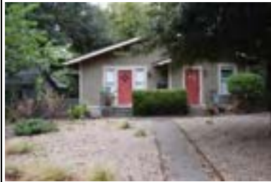
Address: 3212 Oakmont Blvd Year Built: 1948 HHM ID: 96470 NR Recommendation: Update previous district listing
