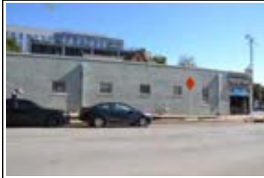
Address: 510 W M L King Jr Blvd Year Built: 1921 HHM ID: 111315 NR Recommendation: Individually eligible
