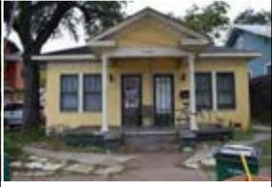
Address: 2902 West Ave Year Built: 1931 HHM ID: 109015 NR Recommendation: Within district
