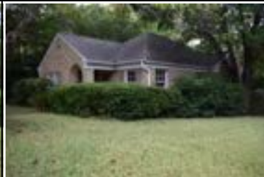
Address: 3106 Beverly Rd Year Built: 1940 HHM ID: 96189 NR Recommendation: Maintain previous district listing
