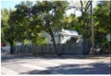
Address: 3213 Kerbey Ln Year Built: 1941 HHM ID: 98488 NR Recommendation: Update previous district listing
