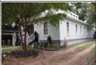
Address: 4302 Avenue A Year Built: 1920 HHM ID: 103422 NR Recommendation: Individually eligible, Within district
