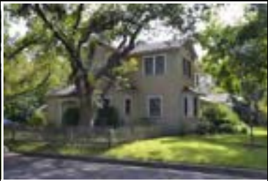
Address: 3211 Glenview Ave (A) Year Built: 1940 HHM ID: 98054 NR Recommendation: Update previous district listing
