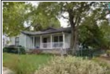
Address: 601 E 47 St (A) Year Built: 1948 HHM ID: 97344 NR Recommendation: Within district
