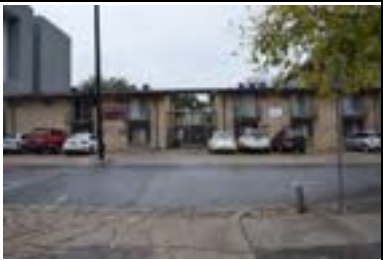
Address: 2612 Salado St Year Built: 1965 HHM ID: 110583 NR Recommendation: Not eligible
