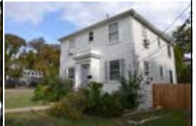
Address: 3211 Tom Green St Year Built: 1940 HHM ID: 107798 NR Recommendation: Within district
