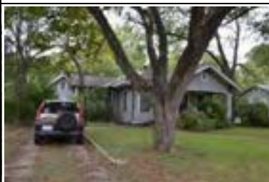
Address: 4706 Rowena St Year Built: 1925 HHM ID: 97911 NR Recommendation: Within district
