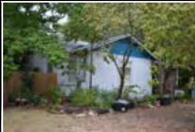
Address: 4804 Red River St Year Built: 1948 HHM ID: 96807 NR Recommendation: Within district
