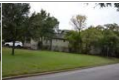
Address: 2902 Hemphill Park (A) Year Built: 1930 HHM ID: 108909 NR Recommendation: Individually eligible
