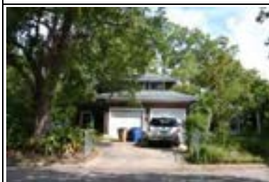
Address: 4512 Caswell Ave (B) Year Built: 1960 HHM ID: 97282 NR Recommendation: Within district
