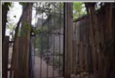
Address: 2910 Fruth St (C) Year Built: 1936 HHM ID: 108638 NR Recommendation: Not able to determine based on visibility
