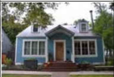
Address: 4510 Avenue B (A) Year Built: 1936 HHM ID: 103694 NR Recommendation: Within district
