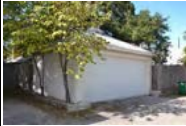
Address: 2847 Shoal Crest Ave (B) Year Built: 1931 HHM ID: 109656 NR Recommendation: Within district
