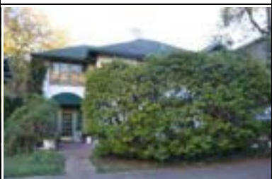
Address: 909 W 23 St (A) Year Built: 1925 HHM ID: 111225 NR Recommendation: Individually eligible
