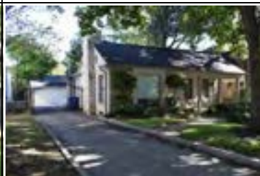
Address: 1504 W 29 St (A) Year Built: 1938 HHM ID: 98854 NR Recommendation: Maintain previous district listing
