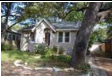
Address: 2837 Shoal Crest Ave (A) Year Built: 1936 HHM ID: 109760 NR Recommendation: Within district
