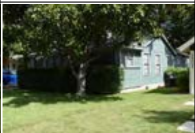
Address: 3305 Bryker Dr Year Built: 1941 HHM ID: 96100 NR Recommendation: Maintain previous district listing
