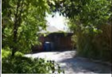
Address: 1901 Cliff St Year Built: 1955 HHM ID: 110693 NR Recommendation: Maintain previous listing, Within district
