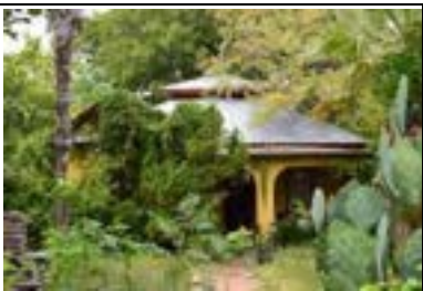
Address: 4714 Rowena St Year Built: 1925 HHM ID: 97888 NR Recommendation: Within district
