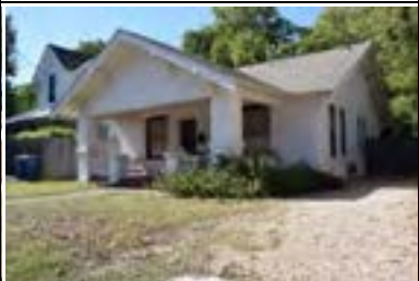
Address: 3310 Jefferson St Year Built: 1920 HHM ID: 98452 NR Recommendation: Maintain previous district listing
