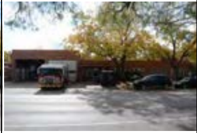
Address: 201 W 30 St Year Built: 1956 HHM ID: 111516 NR Recommendation: Individually eligible
