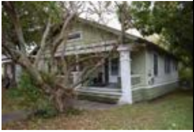
Address: 611 W 31 1/2 St Year Built: 1920 HHM ID: 109179 NR Recommendation: Individually eligible, Within district
