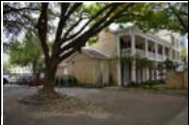
Address: 2620 Rio Grande St (A) Year Built: 1871 HHM ID: 110443 NR Recommendation: Individually eligible
