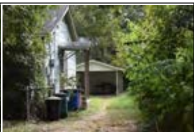
Address: 701 E 50 St (C) Year Built: 1951 HHM ID: 97450 NR Recommendation: Within district
