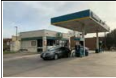
Address: 3515 N Lamar Blvd Year Built: 1965 HHM ID: 113317 NR Recommendation: Not eligible
