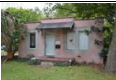
Address: 5005 Avenue G (A) Year Built: 1937 HHM ID: 98001 NR Recommendation: Within district
