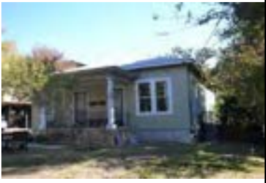
Address: 1909 Cliff St (A) Year Built: 1925 HHM ID: 111271 NR Recommendation: Within district
