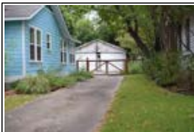
Address: 508 E 49 St (B) Year Built: 1951 HHM ID: 97752 NR Recommendation: Within district
