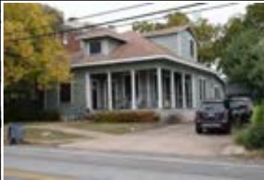
Address: 110 E 30 St (A) Year Built: 1916 HHM ID: 108497 NR Recommendation: Within district
