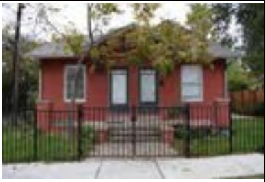
Address: 2900 West Ave Year Built: 1932 HHM ID: 109006 NR Recommendation: Within district
