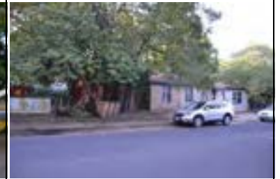
Address: 1700 W 32 St Year Built: 1952 HHM ID: 98139 NR Recommendation: Update previous district listing
