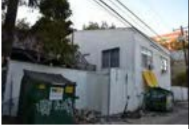
Address: 2305 Nueces St (B) Year Built: 1920 HHM ID: 111413 NR Recommendation: Not eligible
