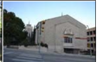
Address: 1909 University Ave (A) Year Built: 1960 HHM ID: 111205 NR Recommendation: Individually eligible
