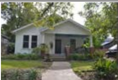
Address: 4803 Avenue F (A) Year Built: 1930 HHM ID: 97735 NR Recommendation: Individually eligible, Within district
