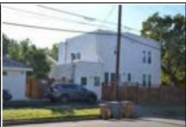
Address: 400 E 34 St Year Built: 1927 HHM ID: 105063 NR Recommendation: Individually eligible, Within district
