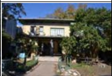
Address: 710 W 21 St Year Built: 1931 HHM ID: 111268 NR Recommendation: Individually eligible
