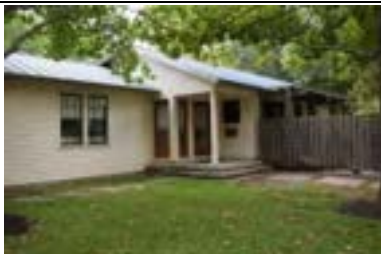
Address: 3401 Oakmont Blvd Year Built: 1947 HHM ID: 95892 NR Recommendation: Maintain previous district listing
