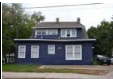
Address: 1100 W 22 St (A) Year Built: 1916 HHM ID: 110135 NR Recommendation: Within district
