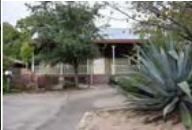
Address: 4522 Avenue G Year Built: 1894 HHM ID: 103015 NR Recommendation: Individually eligible, Within district
