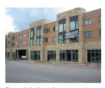
**Figure 5-3:** Shows façade articulation with a change in plane and also change in color and material.
