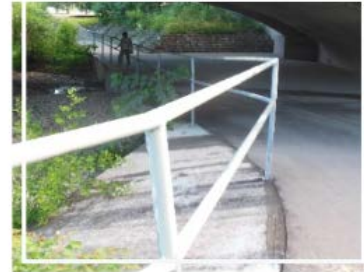
Large Gaps in Handrails
