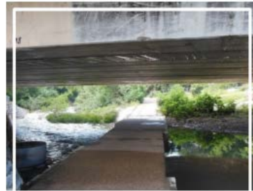
Missing Handrails
